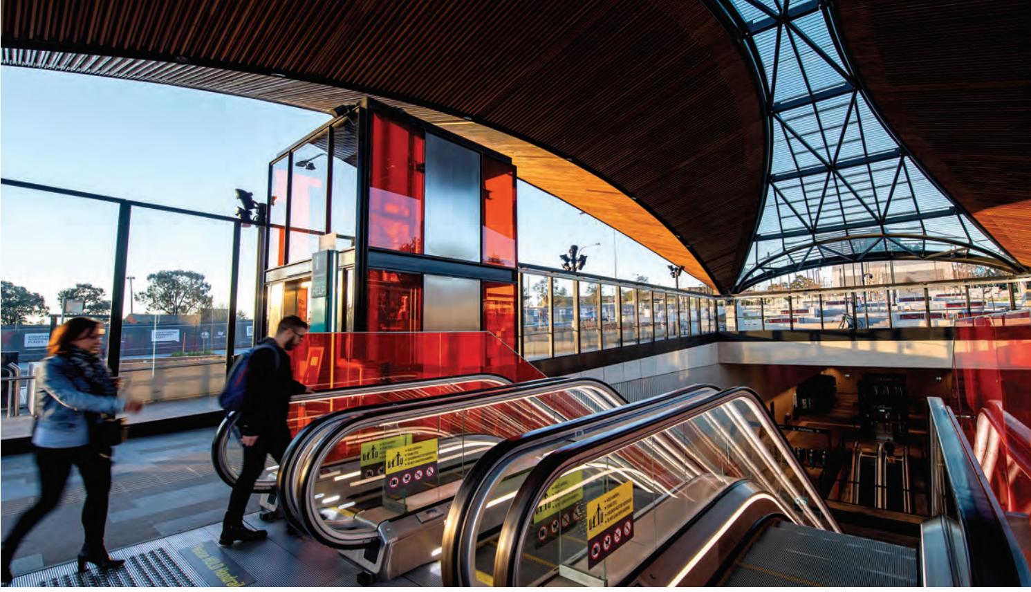
Hills Showground Station, Metro North West Line.
