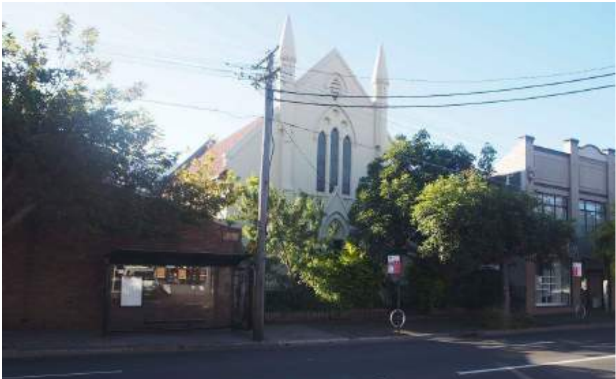
Figure 26 – View of Waterloo Congregational Church from Botany Road prior to demolition of adjacent lands
