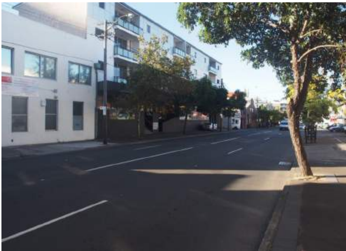
Figure 28 – View facing south on Botany Road pre-demolition
