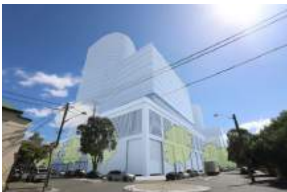
Viewpoint 4 – Corner Cope Street and Wellington Street, facing north-west
