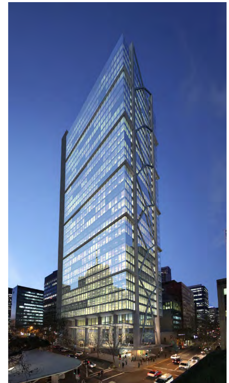
100 MOUNT STREET / SOM AND ARCHITECTUS/ UNDER CONSTRUCTION
