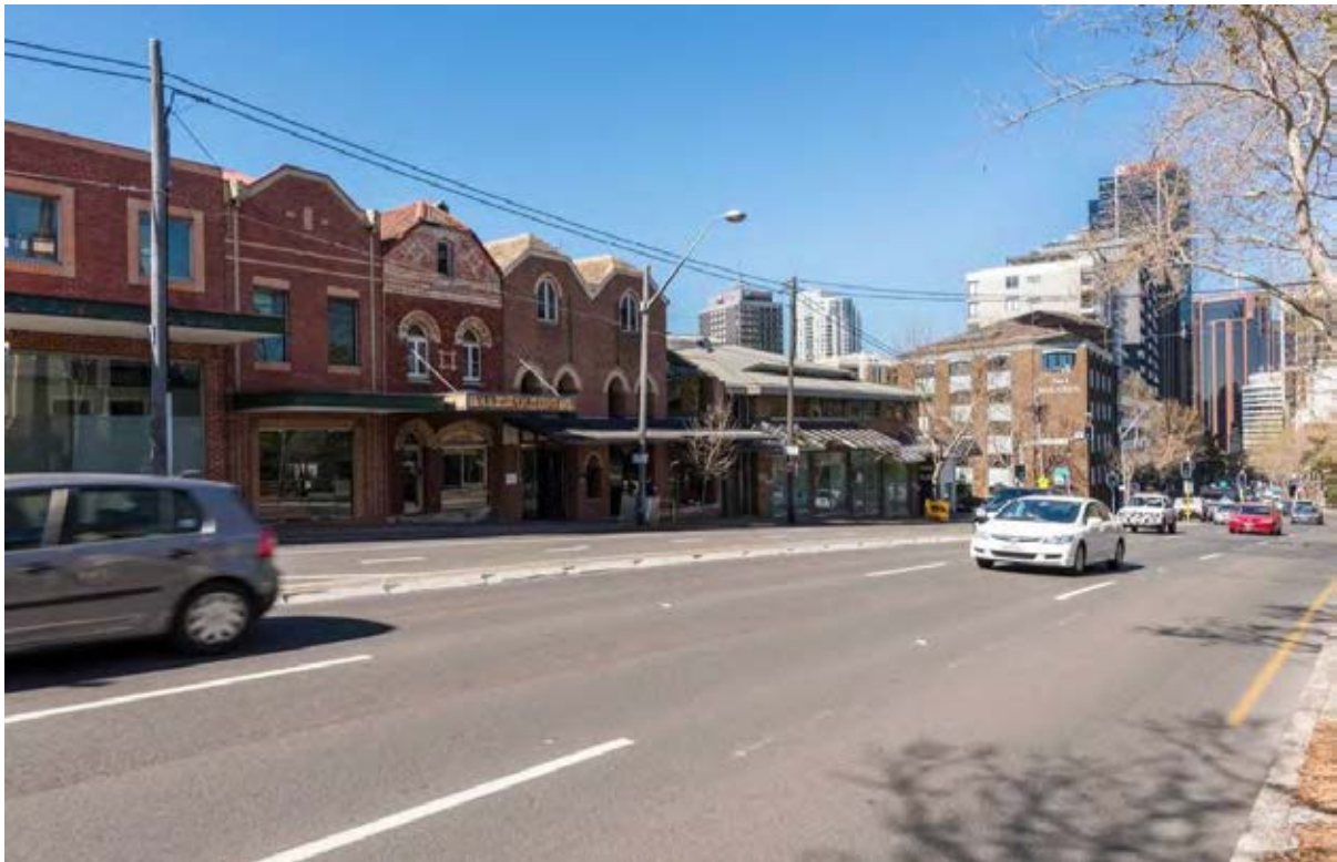
Figure 25: Viewpoint 8: Corner of West Street and Pacific Highway, North Sydney, existing view
