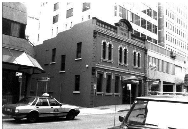
Figure 34: Former Fire Station. Source: State Heritage Inventory Listing Sheet
