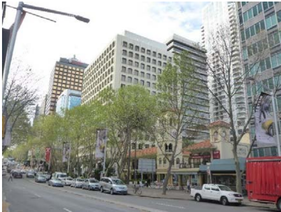
Figure 19: View looking north along Miller Street in 2016, prior to the commencement of demolition works, showing Tower Square on the southern end of the subject site and the mid-rise commercial office building at 181 Miller Street. Source: OCP Architects, 2016
