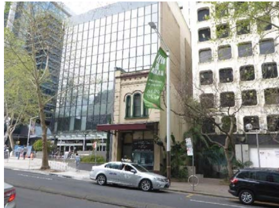
Figure 20: View of the subject site in 2016, prior to the commencement of demolition works, showing the Victorian Shop at 187 Miller Street. Source: OCP Architects, 2016
