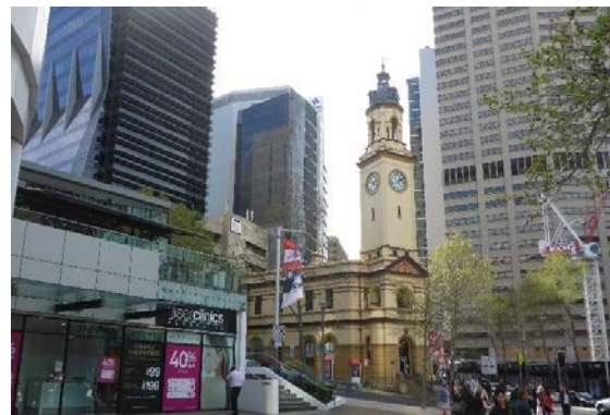
Figure 17: View of the North Sydney Post Office building on the corner of Miller Street and the Pacific Highway. Source: OCP Architects, 2016
