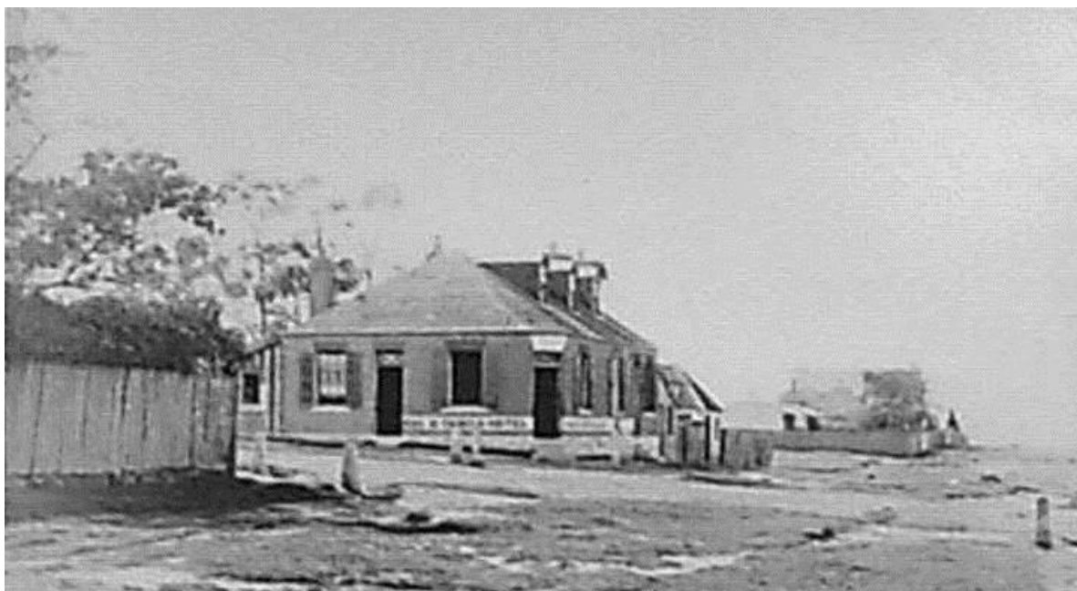
Figure 10: The Rag & Famish Hotel on Berry Street in c.1860. Source: The Face of North Sydney photo archives, LH REF PF851. (Copyright – Mitchell Library)
