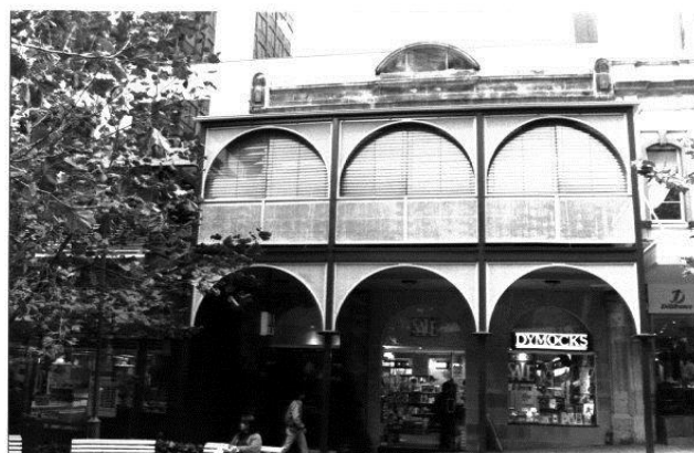
Figure 32: Façade of S Thompson Building. Source: State Heritage Inventory Listing Sheet
