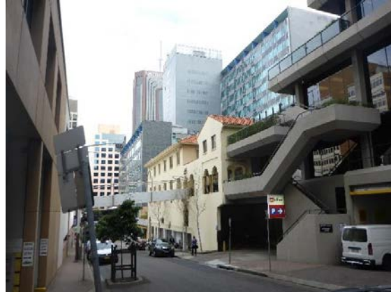
Figure 22: View south along Denison Street showing the rear of the Tower Square shopping centre in 2016, prior to the commencement of demolition works. The rear of the MLC Building is shown in the distance. Source: OCP Architects, 2016
