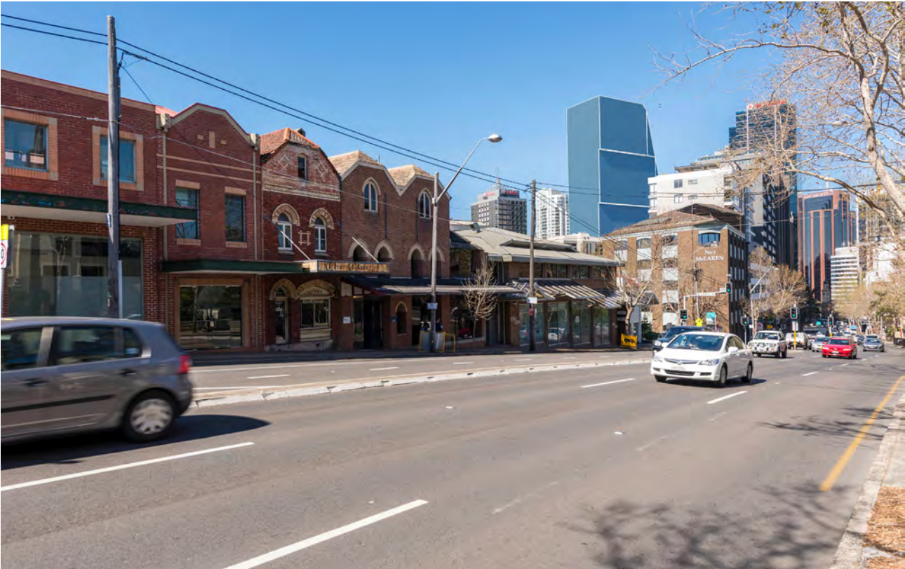
Figure 56 – Envelope seen from intersection McLaren St and Pacific Hwy
