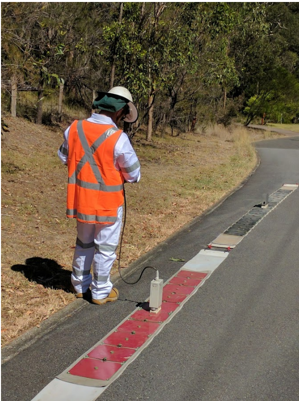
Image 2: DGPR Radar Antenna System
