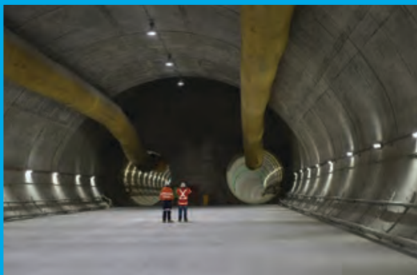
Twin 15-kilometre railway tunnels, Australia's longest at the time of their construction, run from Bella Vista to Epping and include this cavern at Castle Hill.
