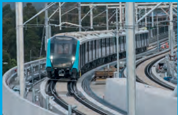
The four-kilometre skytrain viaduct runs from Bella Vista to Rouse Hill and takes the new metro line above the north west, keeping communities connected.
