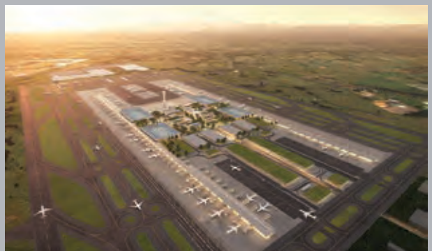
The Australian and NSW governments have a shared objective of having metro rail operational when the Western Sydney International Airport opens for passenger services.
