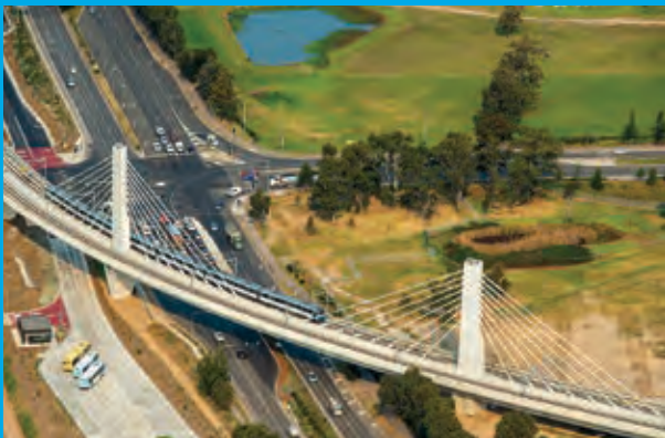
A 270-metre curved cable-stayed bridge at Rouse Hill is the first of its type in Australia and was named global project of the year by US-based Engineering News-Record for its elegant, innovative and sustainable design.
