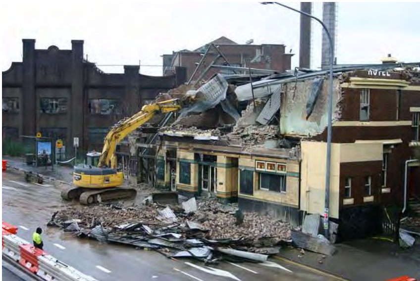
Figure 10: White Bay Hotel under demolition, 2010. 24
