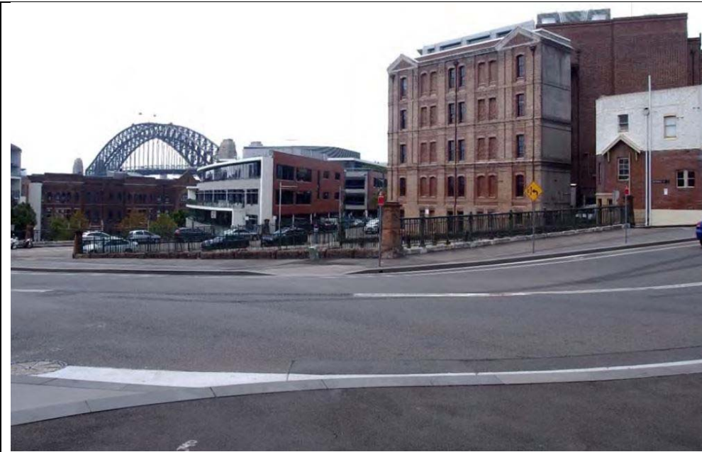
Viewpoint a: View northeast from footpath on Dalgety Road (from Consistency Assessment)
