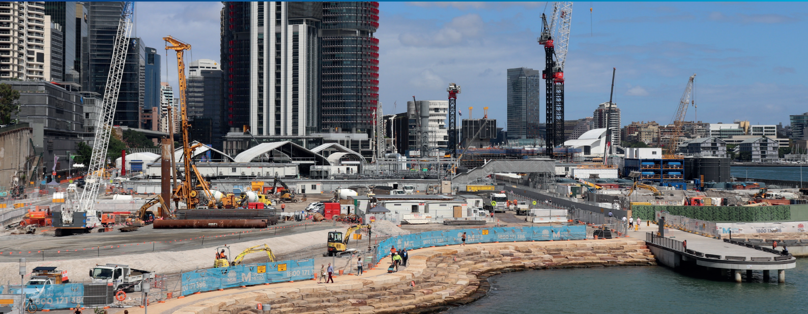
Piling underway at Barangaroo Station site
