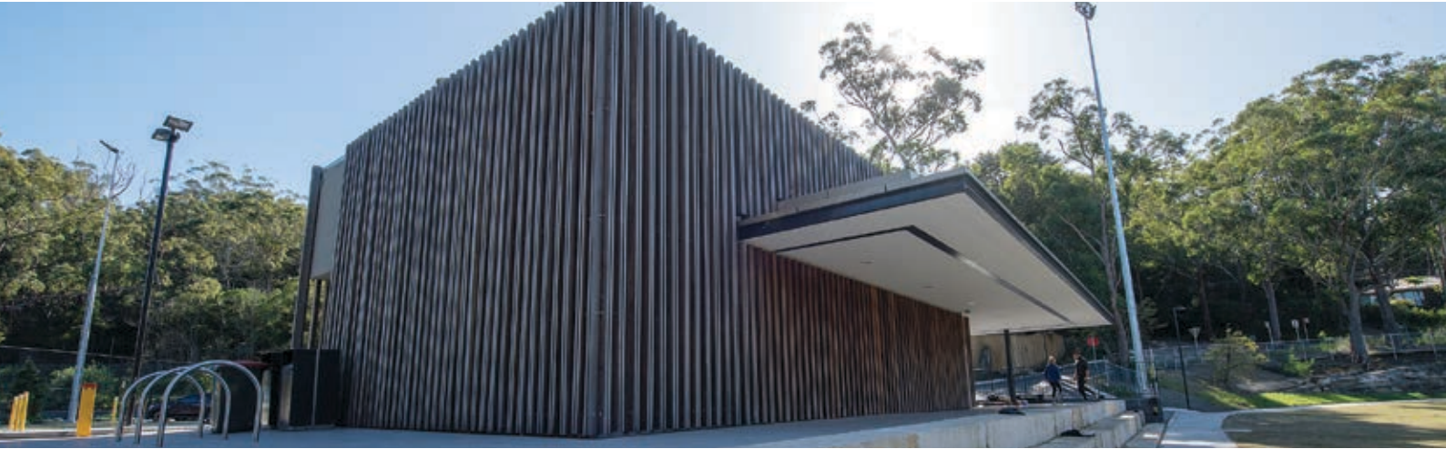
An example of a Sydney Metro services facility at Cheltenham.
