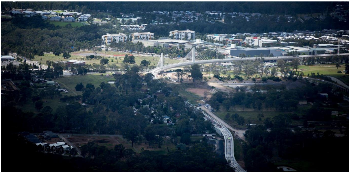
Figure 2 – View of completed Windsor Road Bridge
