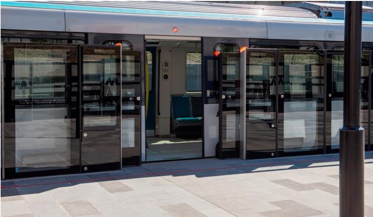
Figure 6 – Testing of Platform Screen Doors at Tallawong
