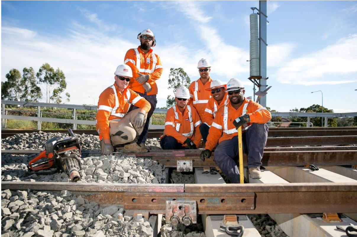
Figure 3 – Installation of the last portion of Sydney Metro Northwest track
