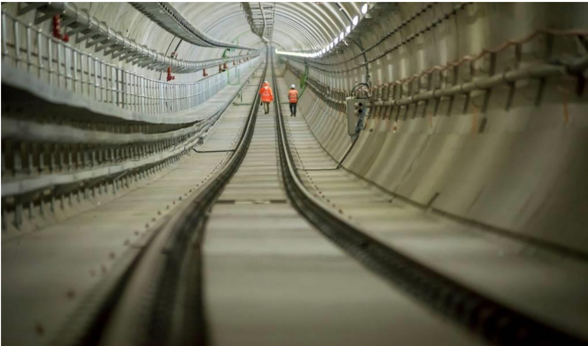
Figure 7 – A look inside the Northwest tunnel
