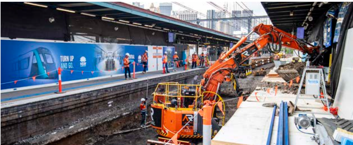
Major construction work at Central Station.
