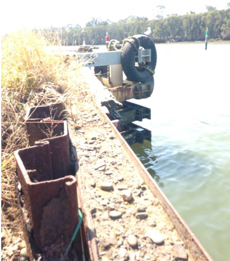
Plate 4.1: Current wharf with Gore Bay pipeline in the background.
