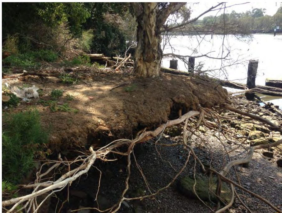
Plate 4.3 Undercutting and erosion of natural banks to the north of the wharf
