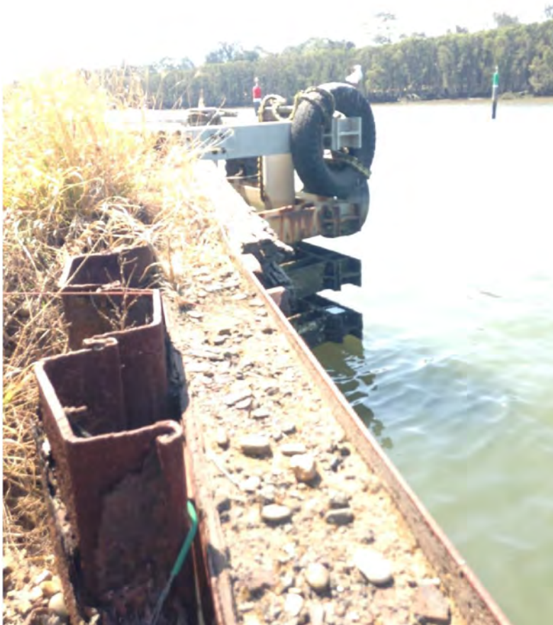
Plate 4.1: Current wharf with Gore Bay pipeline in the background.
