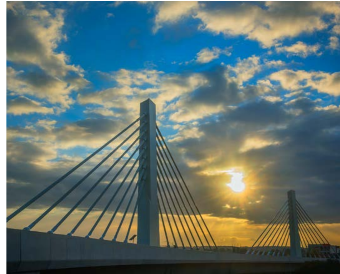
The Windsor Road railway bridge at Rouse Hill.
