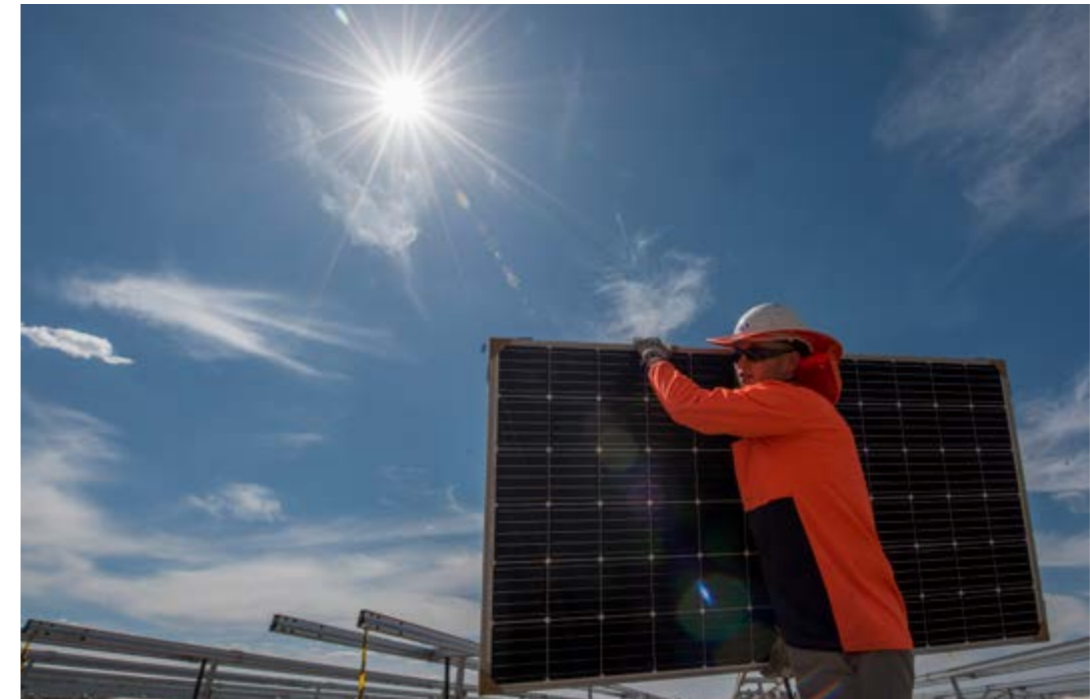
Installation work at the Beryl Solar Farm in regional NSW.
