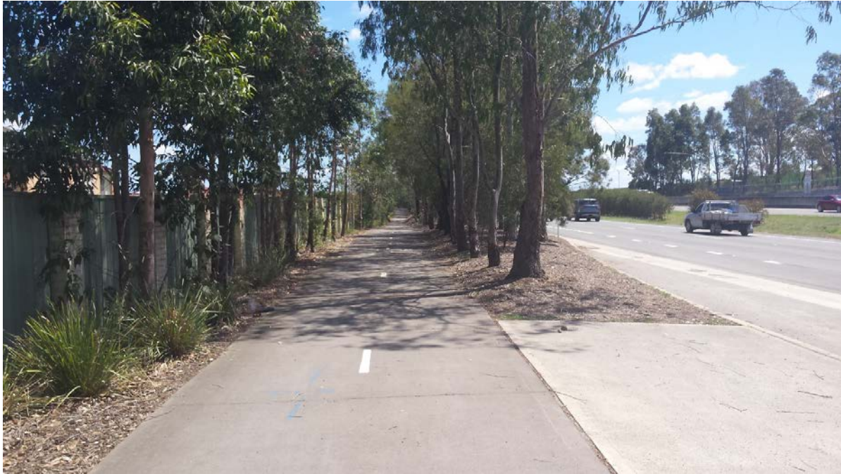
Figure 7-13 View of old Windsor road shared pathway (looking north)
