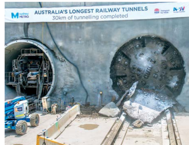
Tunnelling finished on 14 January 2016 with TBM2 Florence's break-through at Cherrybrook
