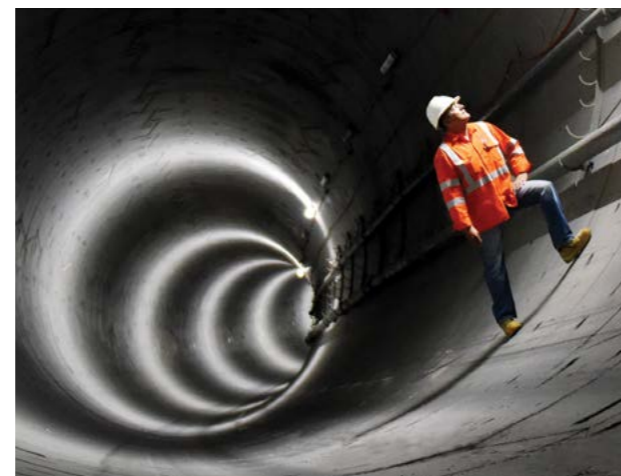
Australia's longest railway tunnels run 15 kilometres from Bella Vista to Epping on Sydney Metro Northwest
