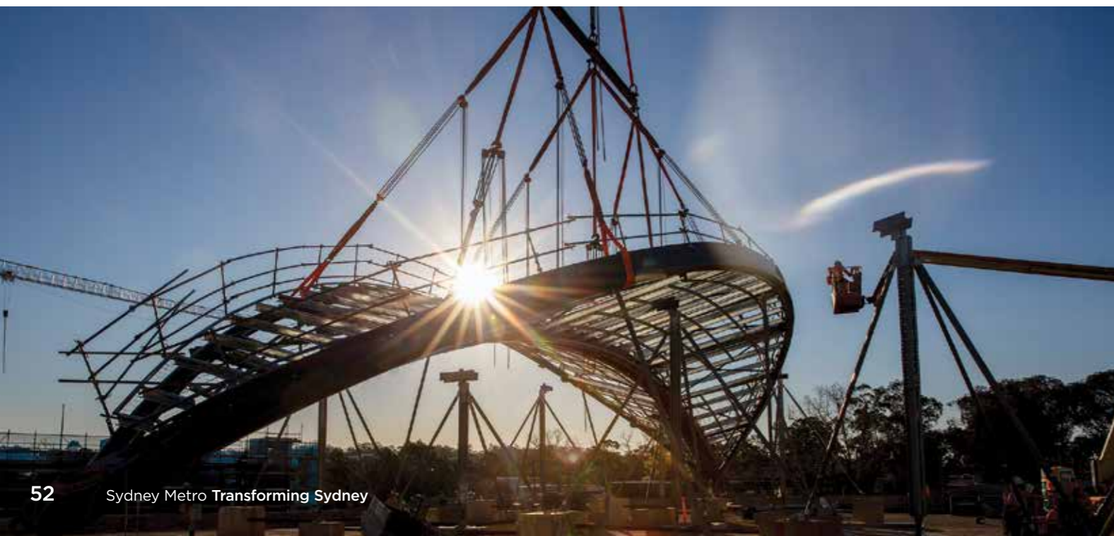
Below: Canopy installation at Hills Showground, October 2018.
