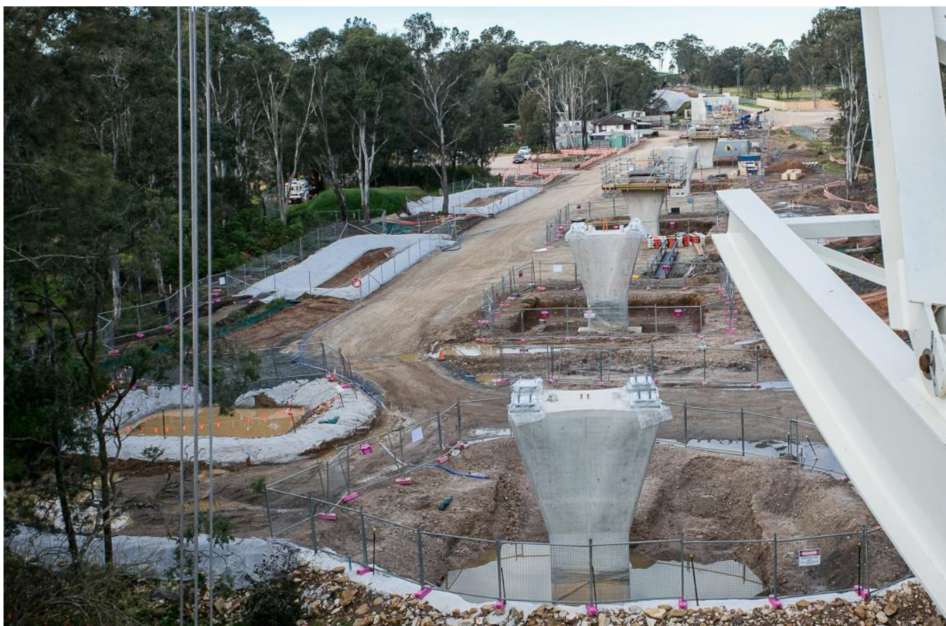
Figure 14 – Erosion and Sediment Controls at the ISJV Cudgegong Road Site
