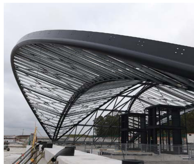
The new Cudgegong Road Station under construction
