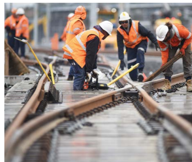
The first railway tracks for Sydney Metro, laid in June 2016
