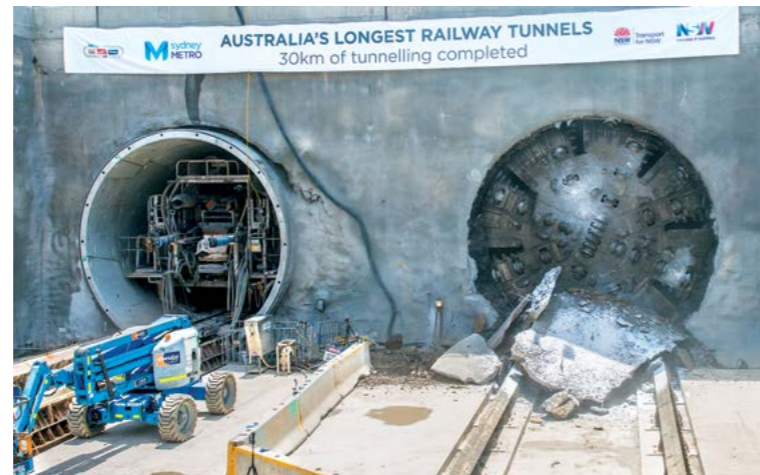
Tunnelling finished on 14 January 2016 with TBM2 Florence's break-through at Cherrybrook
