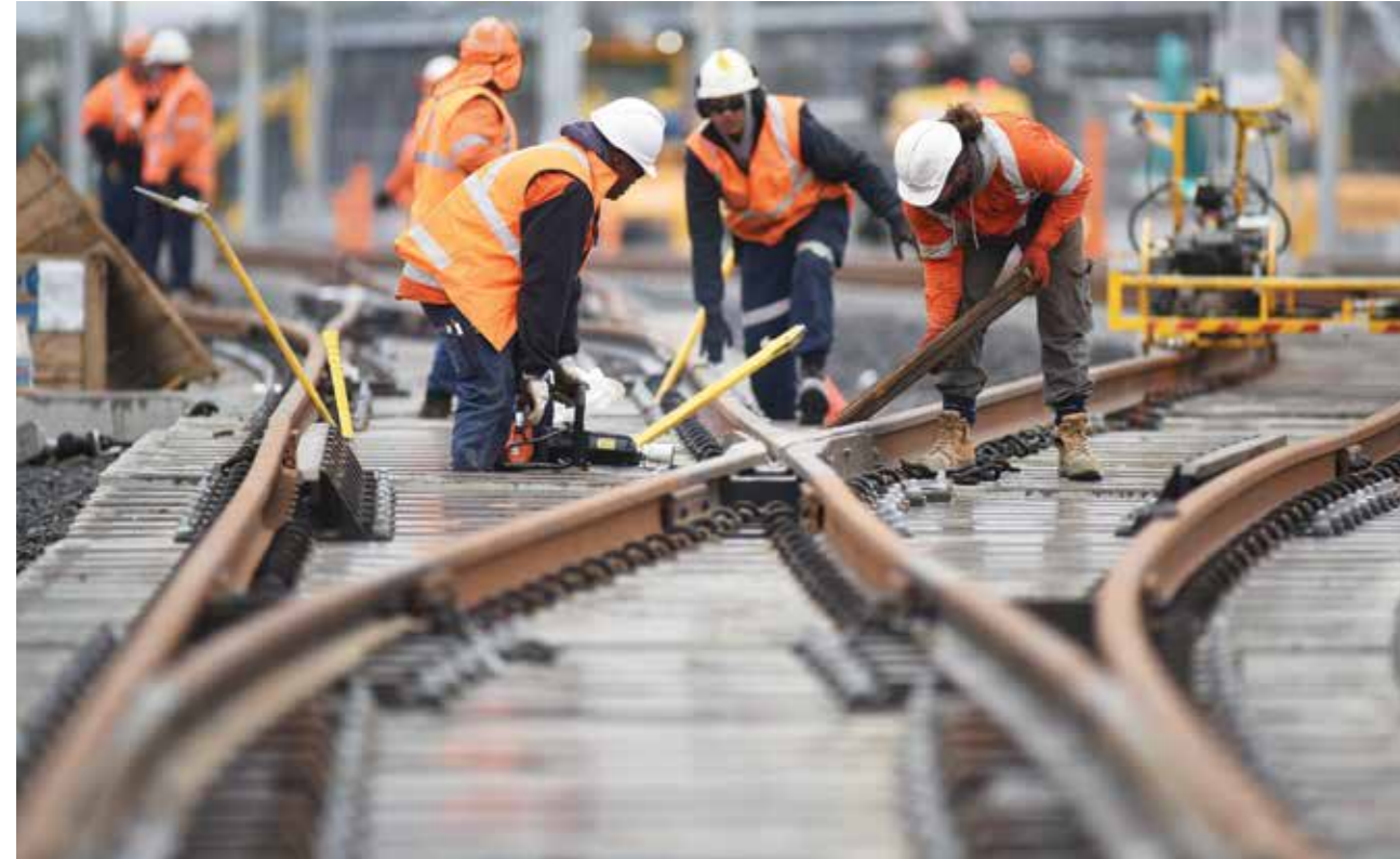
Workers laying tracks at the Sydney Metro Trains Facility, August 2016
