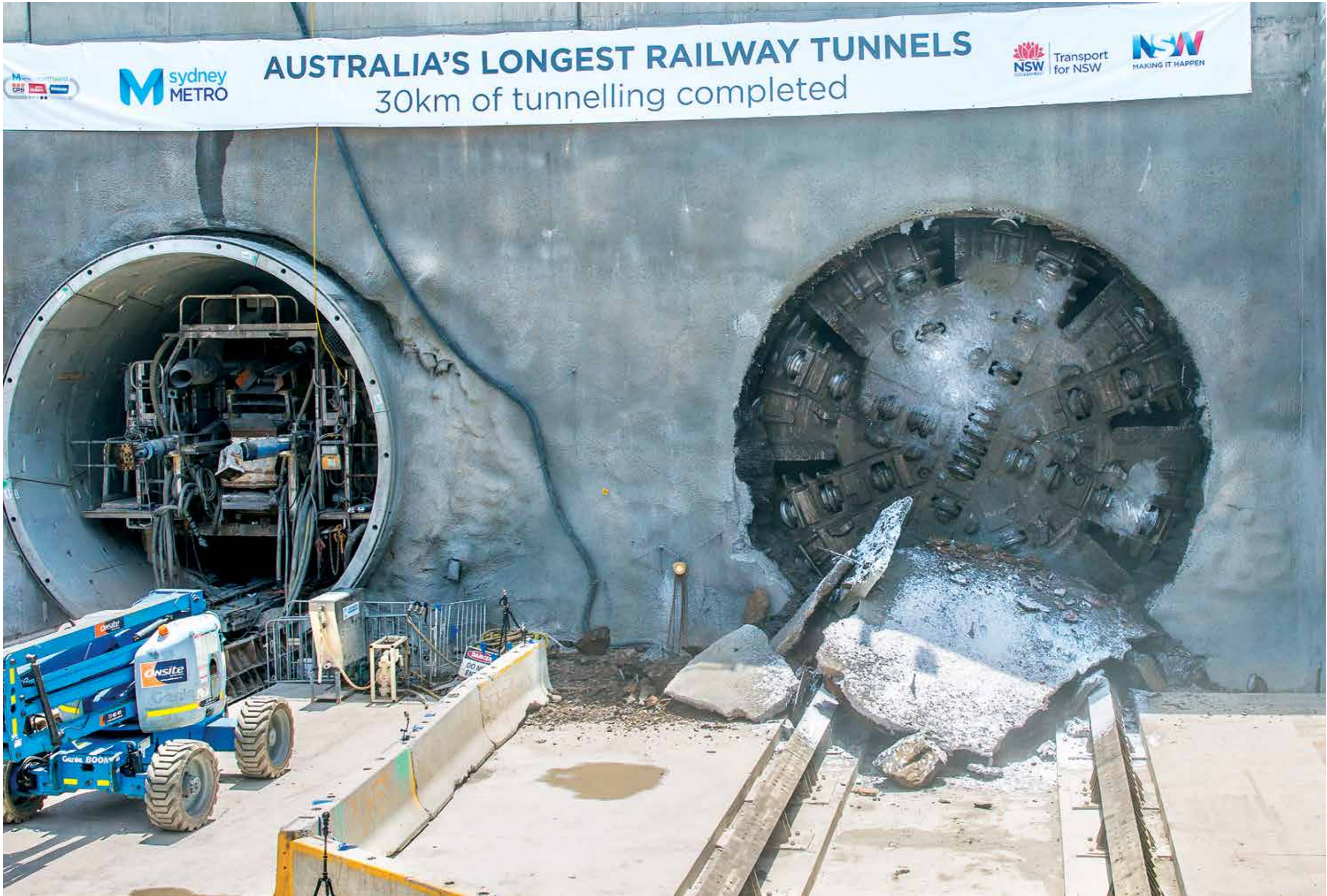
Tunnelling finished on 14 January 2016 with TBM2 Florence's break-through at Cherrybrook
