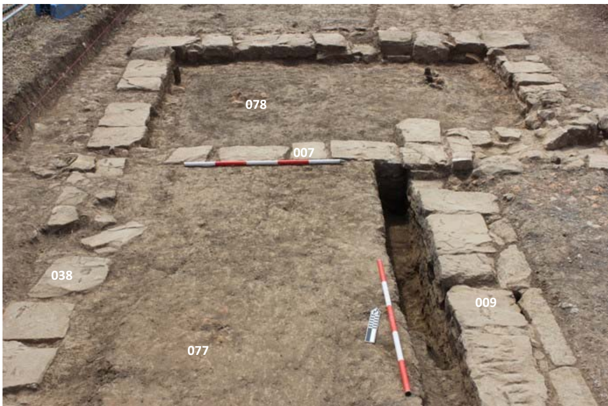
Plate 4.2 The northern extent of the main inn building showing the sondage against the rear veranda footings [009]. View north; scales 1 m each.
