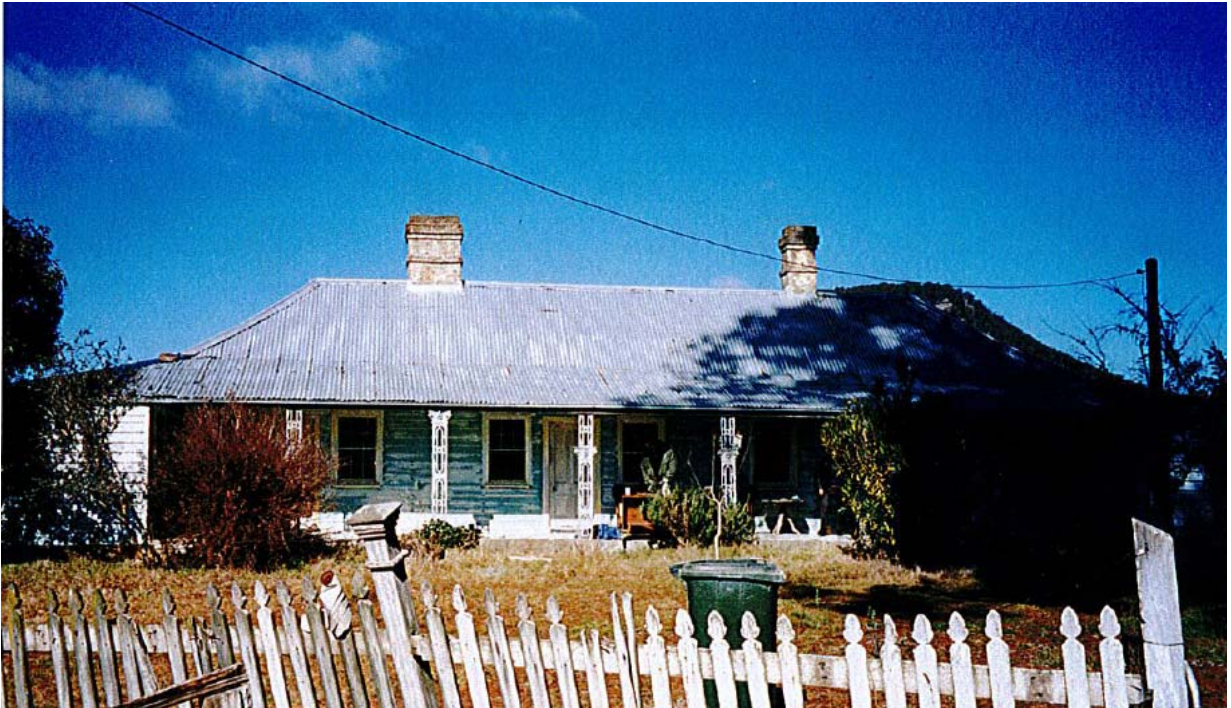
Plate 7.6 Collit's Inn in 2001 prior to restoration works. (Source: Christine and Russell Stewart 2002, Section 4).
