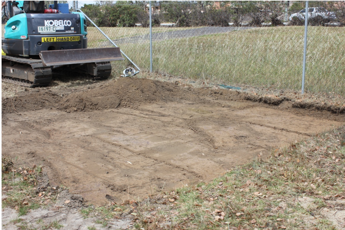
Plate 5.3 Grass and topsoil removal – Stranger’s cottage site. View south-west.
