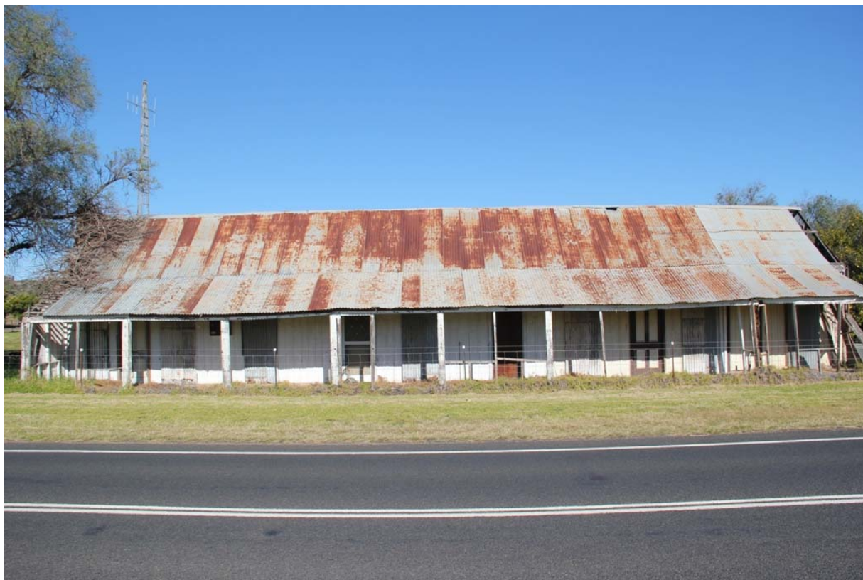
Plate 7.1 An inn on the Narromine Road at Rawsonville (Dubbo LGA).
