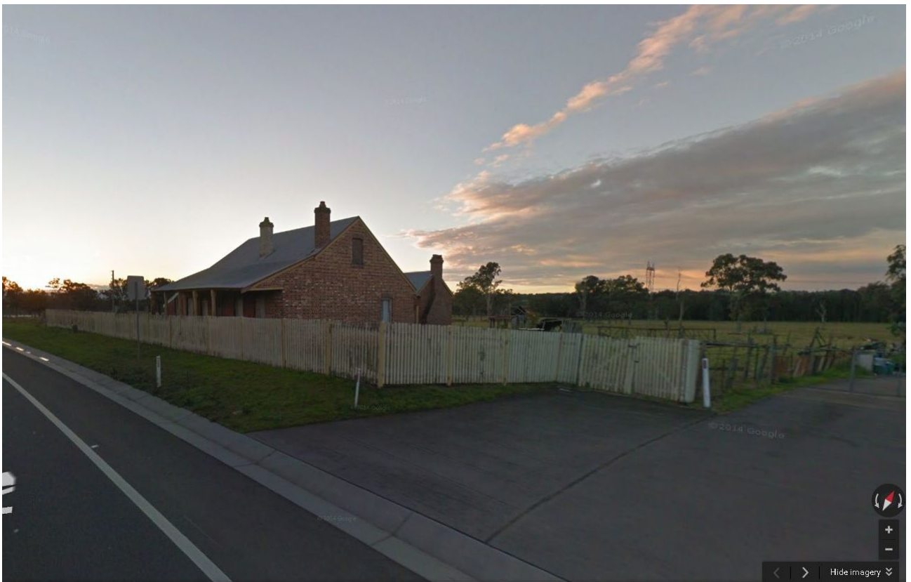
Plate 7.4 Box Hill Inn from Windsor Road. View north east (Source: Google Streetview).
