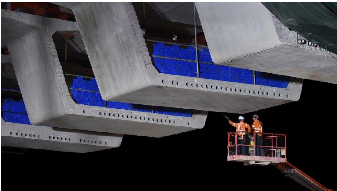
Figure 3 – Final Segment Installation of the Windsor Road Bridge Deck
