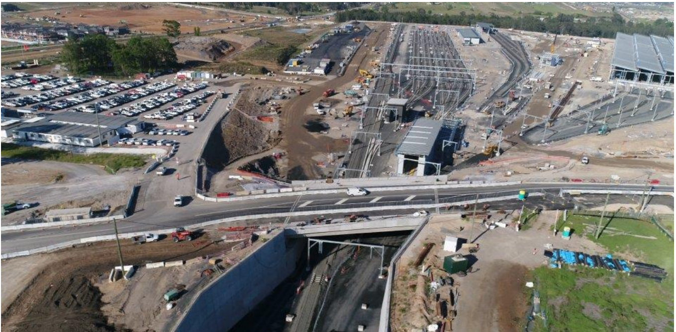
Figure 4 – Tallawong Road Bridge at the SMTF
