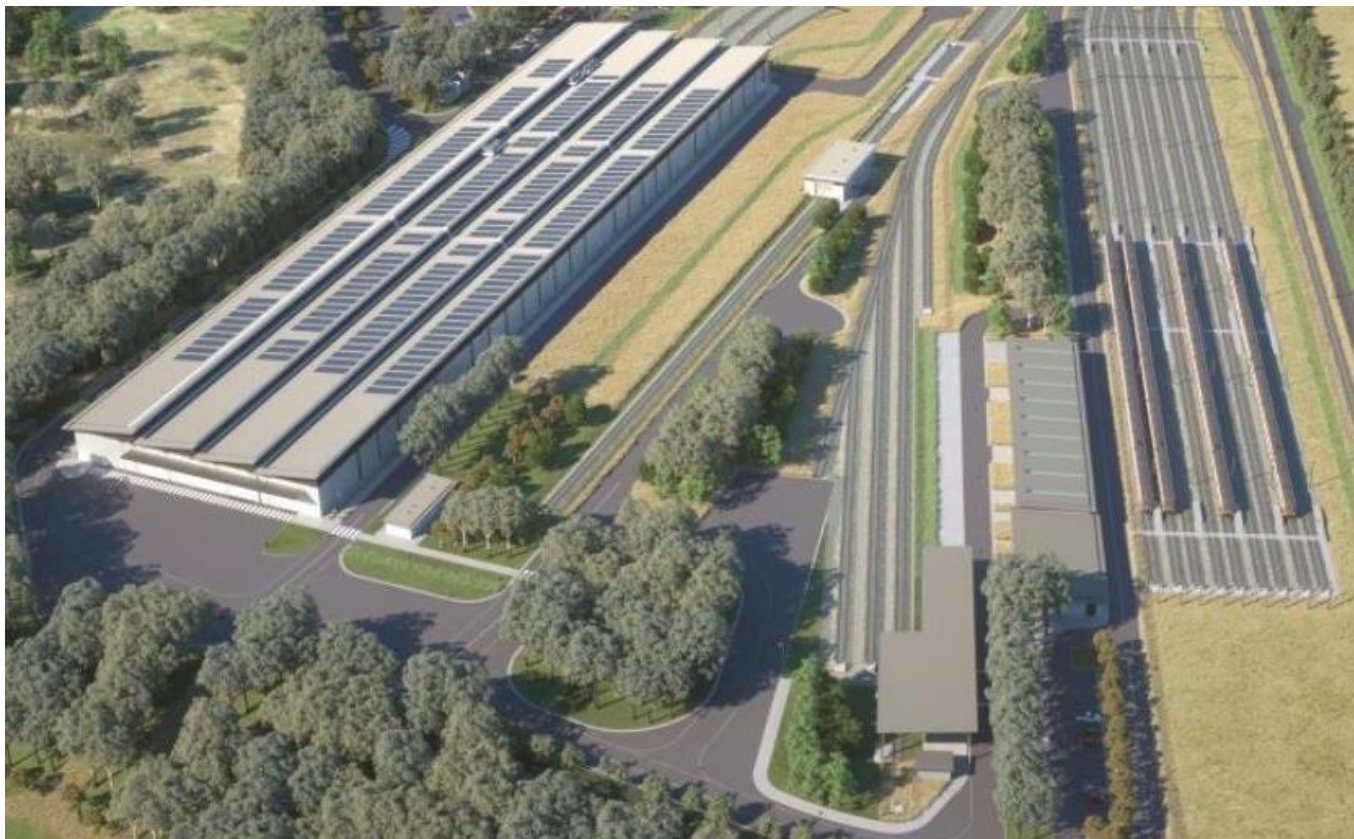
Figure 19 – Artist Impression of the 1.1 MW Solar Photovoltaic System to be installed at the SMTF
