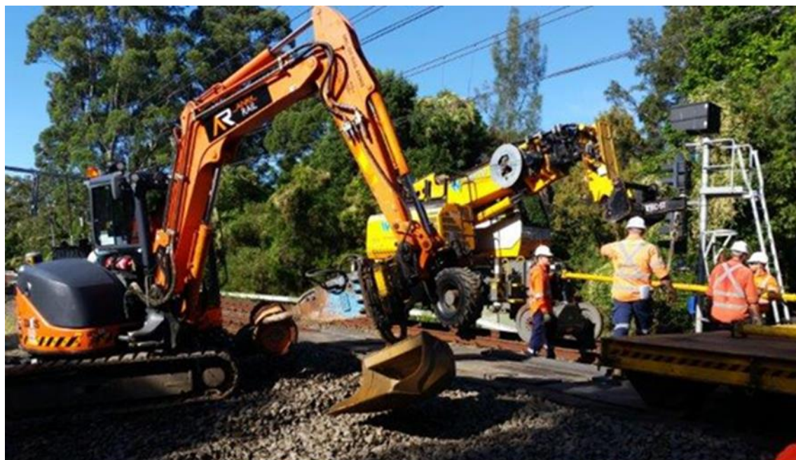
Figure 6 – Weekend possession works along the Northern Corridor being carried out
