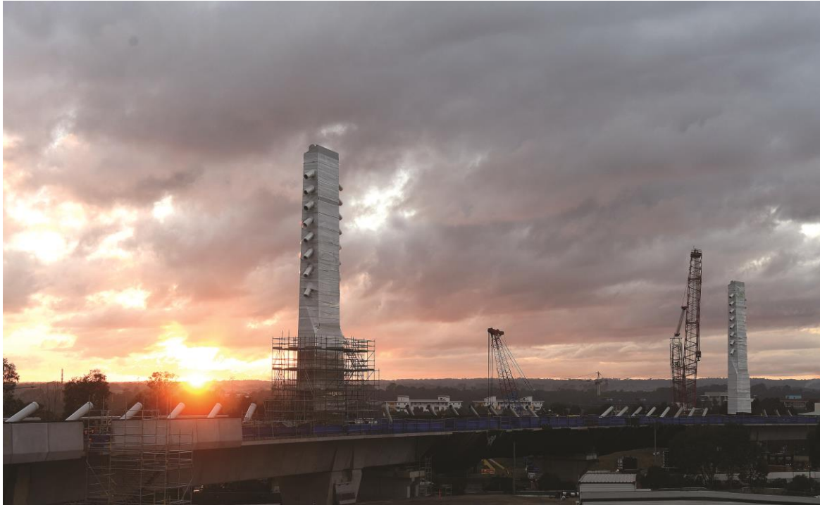
Figure 3 - Windsor Road Bridge under construction
