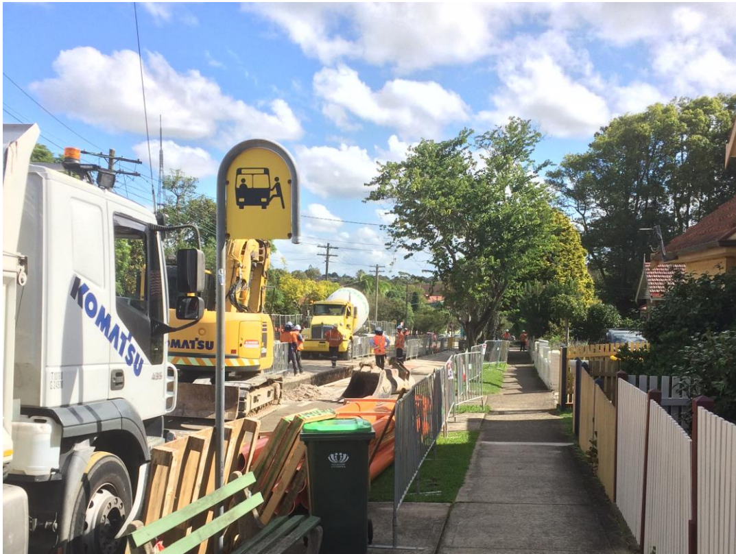
Figure 4 – 33 kV Underground Feeder Powerline works at Hercules Street intersection
