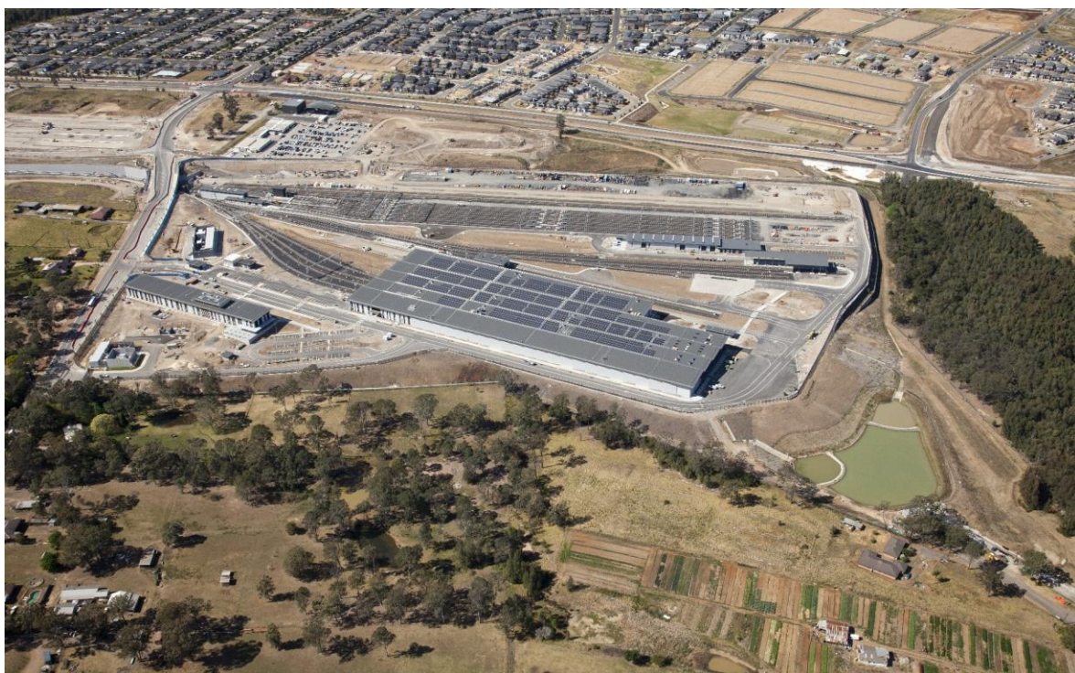
Figure 7 – Aerial view of the Sydney Metro Trains Facility
