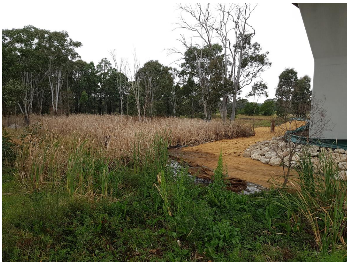
Figure 8 – Landscaping and efforts to protect and enhance waterways under the viaduct
