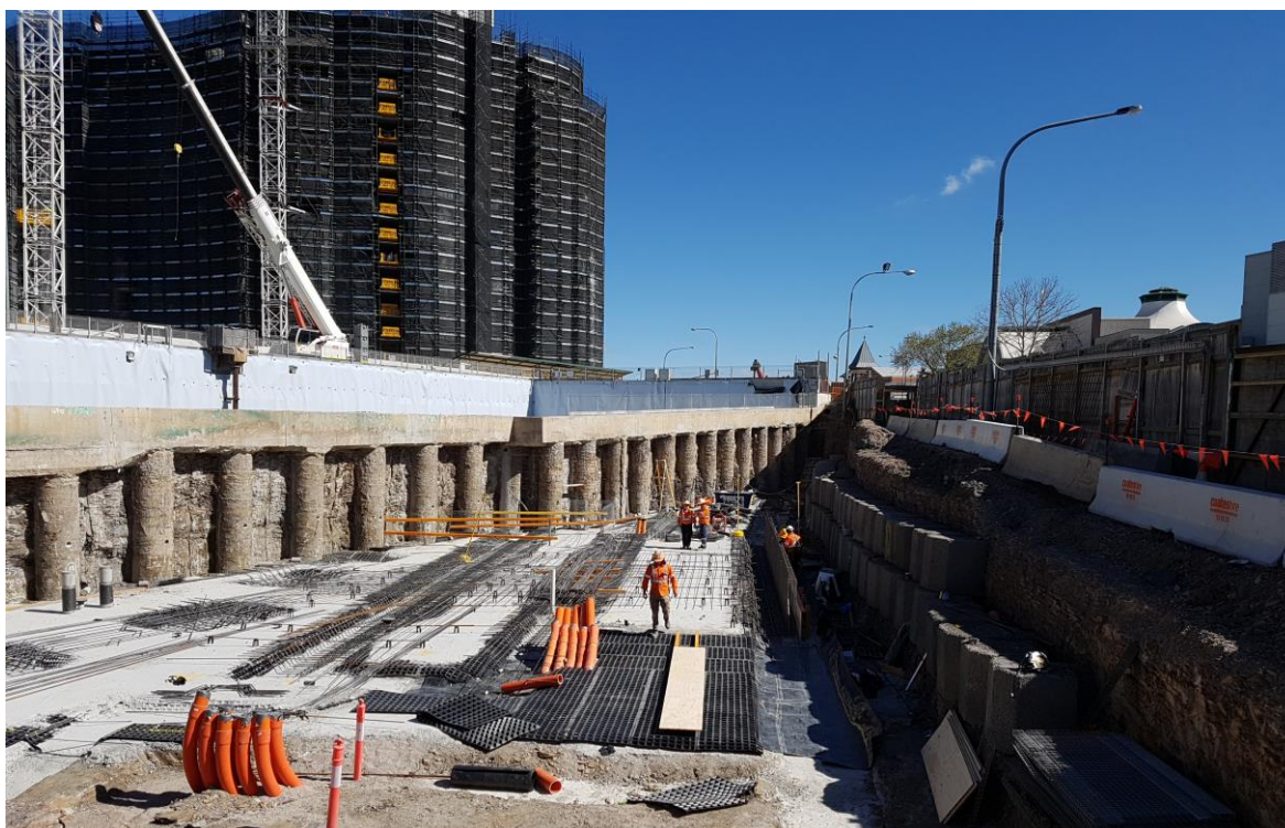
Figure 5 – Work being carried out at the Castle Hill Station box
