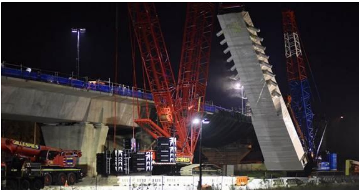
Figure 10 – SVC worksite at the Windsor Road Bridge, night works
