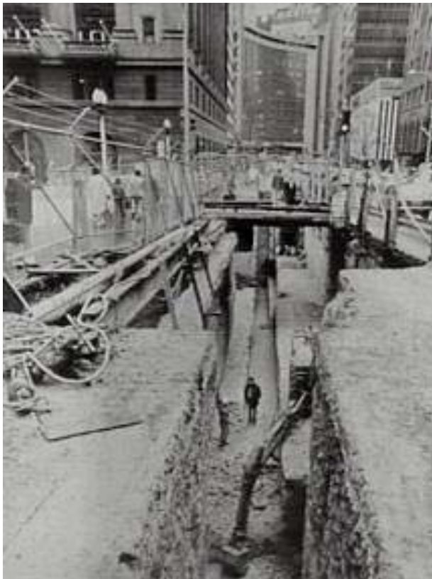
Figure 7-10: Construction of Martin Place Station using open-cut excavation (Source: City of Sydney Archives)
