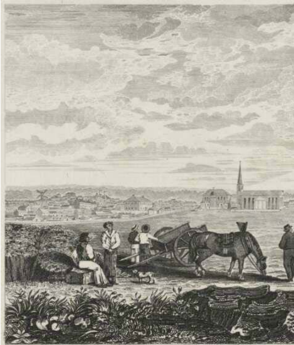
Figure 8-6: Detail of sketch of Sydney, viewed from Hyde Park, 1829. Pitt Street Station site in left background 115
