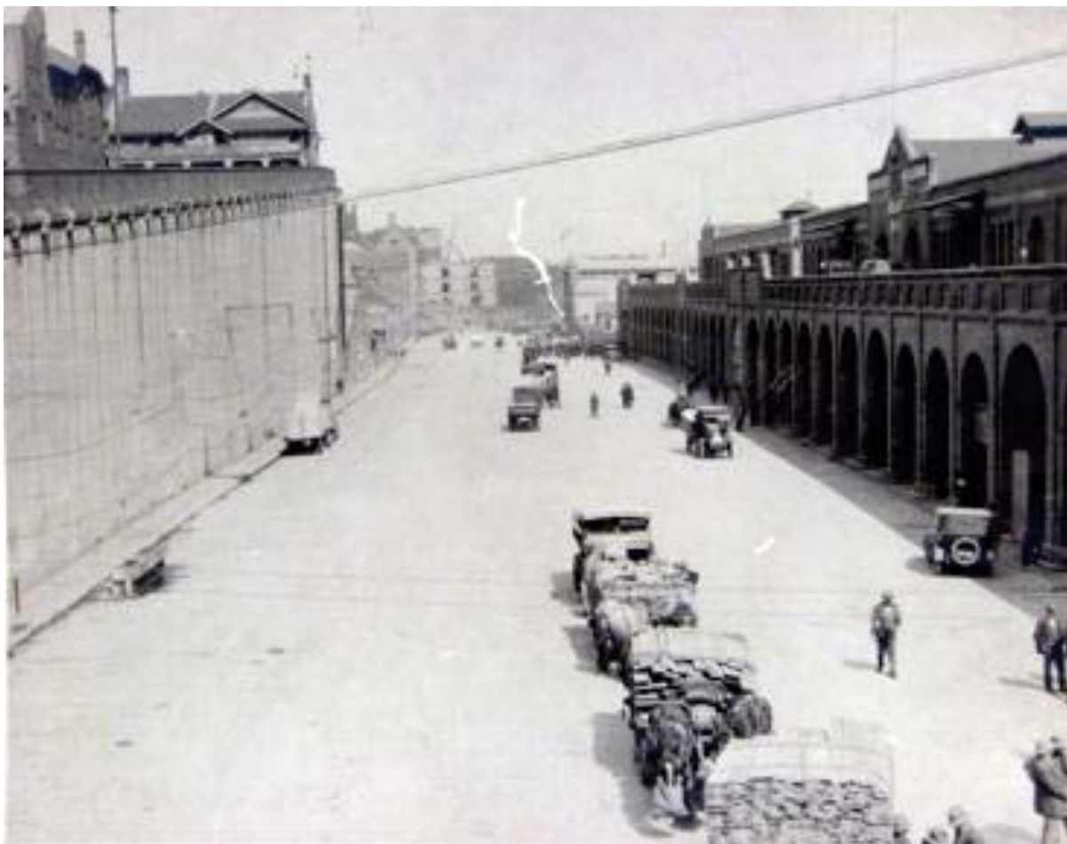
Figure 6-10 View of cutting on Hickson Road and warehouses on the wharf 93
