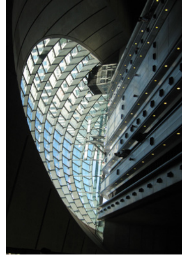
Canary Wharf Station, London. Natural light over entries and VT enhances wayfinding and creates a welcoming station environment. Architect: Foster + Partners Source: Cox Richardson
