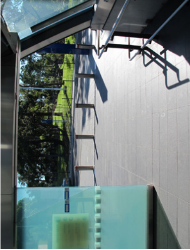
Coordinates interior and exterior public domain pavements. Source: AECOM.
