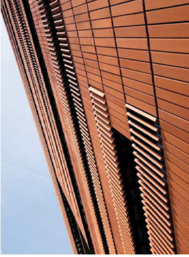
Terracotta louvred facade provides a vibrant wall surface. Source: AECOM.
