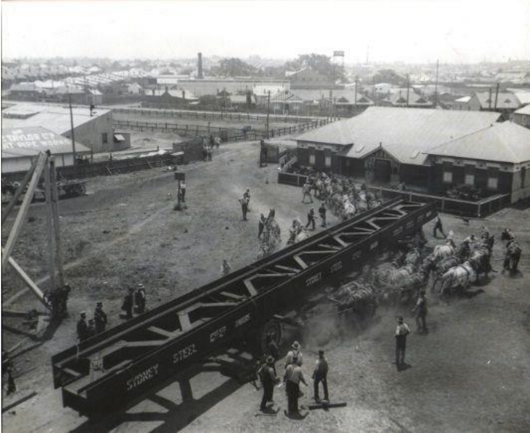
Figure 3-14: Sydney Steel Company, c.1920 [infilled Gumbramorra Swamp area]. Source: Marrickville Council.
