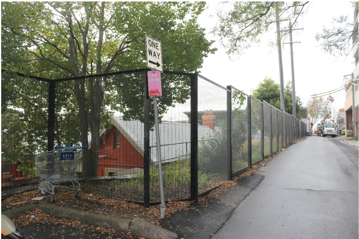
Figure 6-2 View northeast from Lilian Lane
