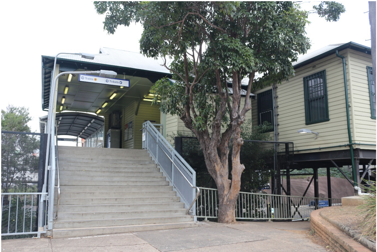
Figure 10-1 View to station entry from Warren Reserve
