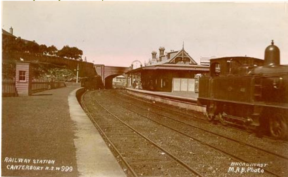
Figure 4-13: n.d. Canterbury Railway Station, showing platforms capping had been removed possibly with the realignment in 1927. Source: ARHS: 023606.
