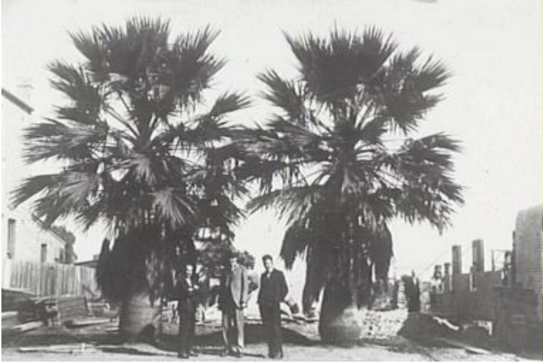
Figure 6-8: Site of the residence of Lakemba after it was demolished. Source: Canterbury City Council.
