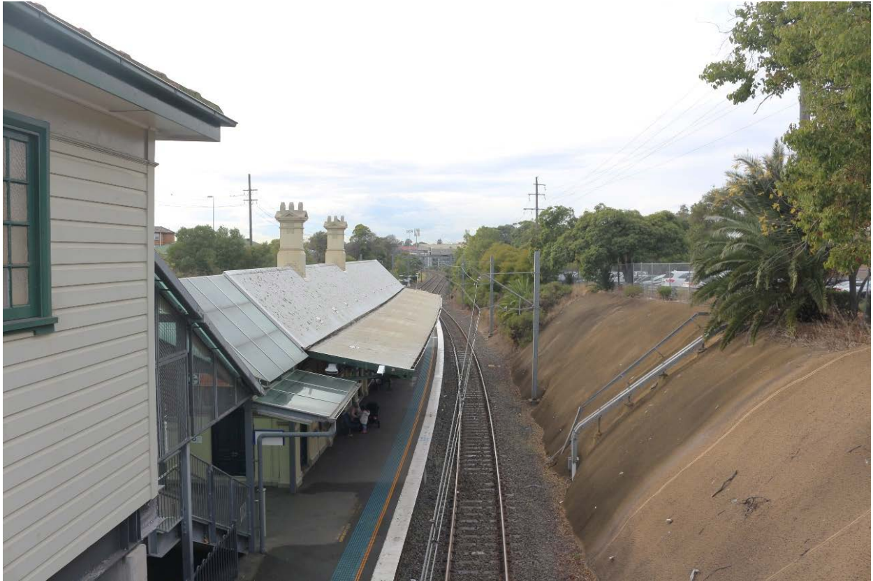
Figure 7-1 View east from Burwood Road overbridge
