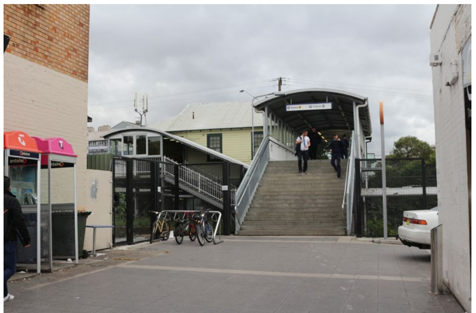
VIEW TO SOUTHERN STATION ENTRY
