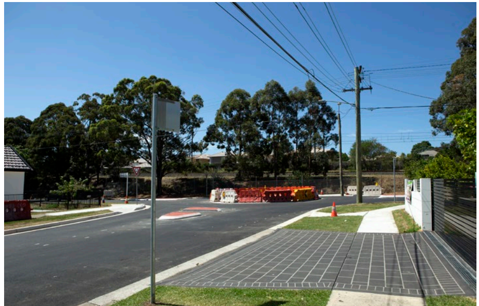
12 VIEW EAST FROM SCOTT STREET
