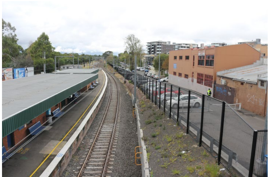
VIEW EAST ALONG THE PUNCHBOWL STATION PLATFORMS
