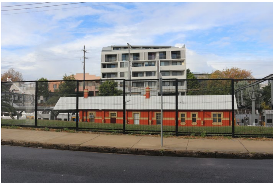
STATION PLATFORM BUILDINGS FROM WILFRED AVENUE
