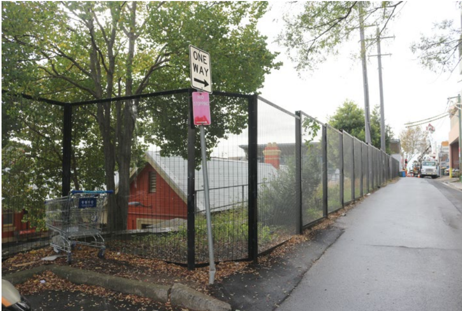
VIEW EAST ALONG LILIAN LANE
