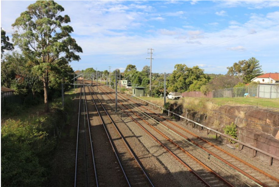
3 VIEW EAST FROM THE MELFORD STREET BRIDGE, BETWEEN HURLSTONE PARK AND CANTERBURY
