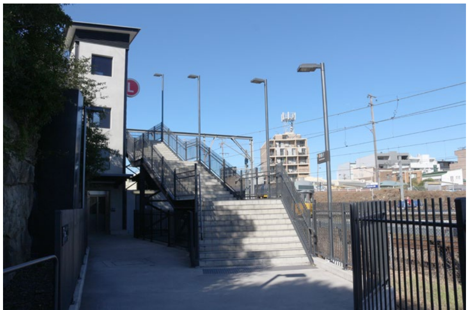
2 VIEW SOUTHEAST FROM DULWICH HILL LIGHT RAIL STATION
