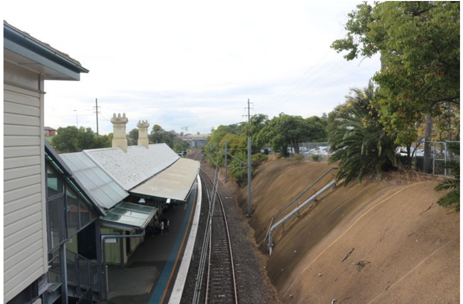
1 VIEW EAST FROM BURWOOD ROAD OVERBRIDGE
