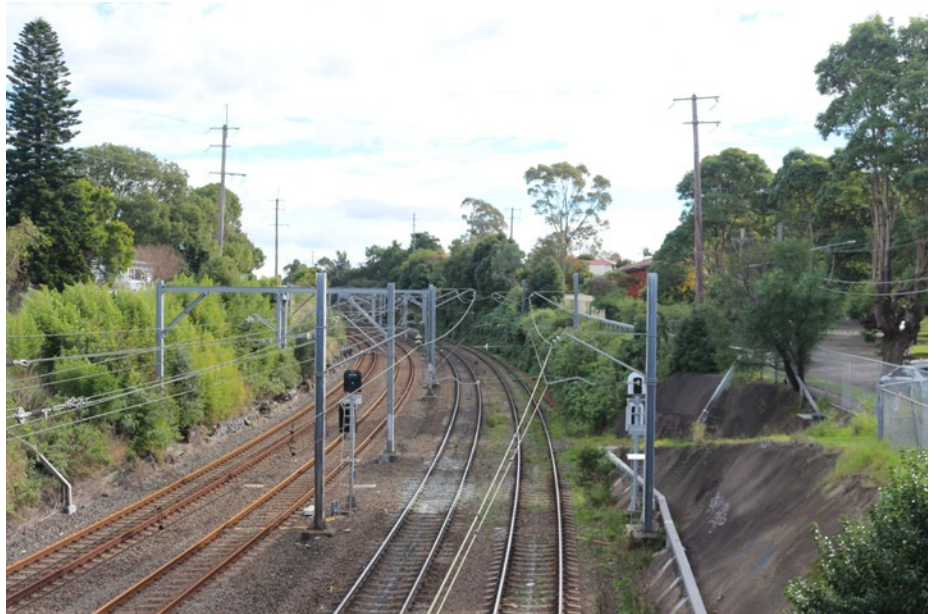
1 VIEW NORTHWEST FROM LIVINGSTONE ROAD, BETWEEN MARRICKVILLE AND DULWICH HILL
