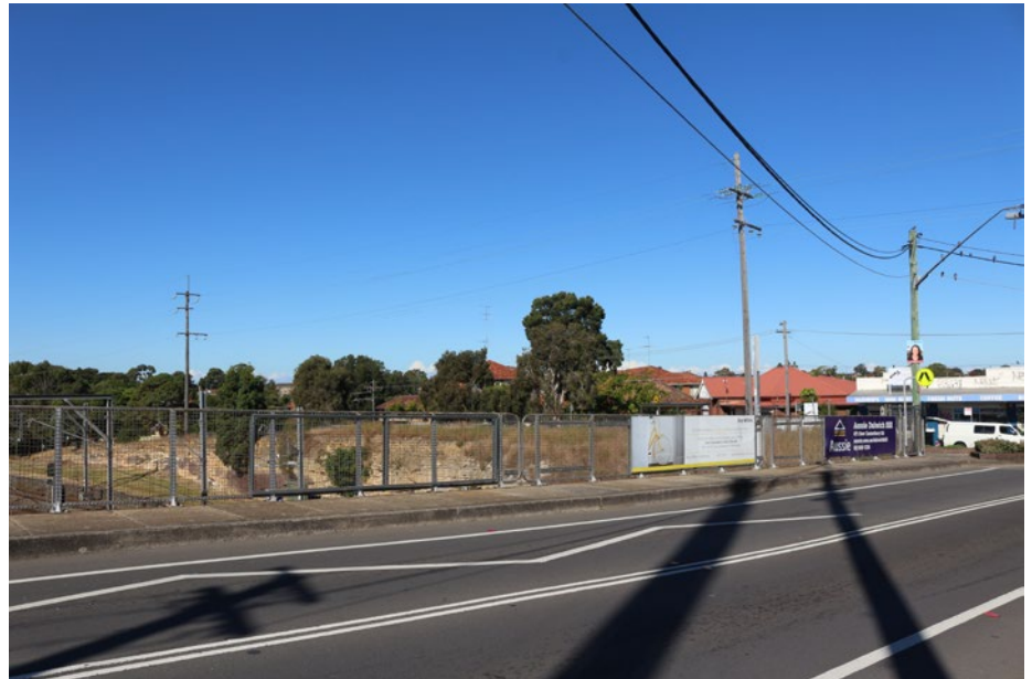
4 VIEW EAST FROM WARDELL ROAD OVERBRIDGE
