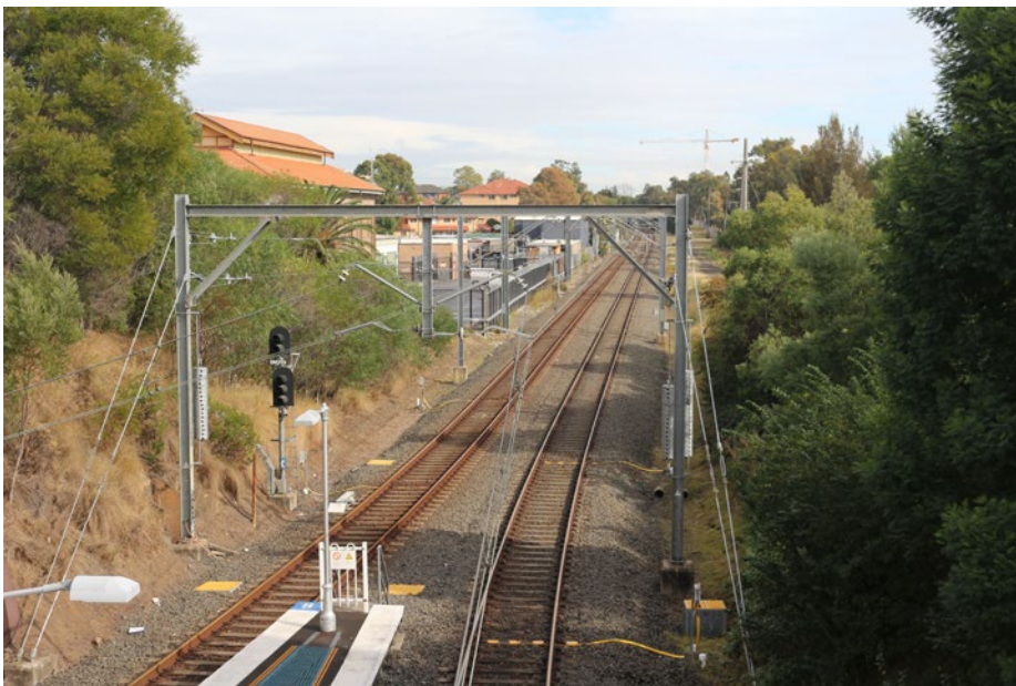
7 VIEW WEST FROM THE BELMORE ROAD BRIDGE, BETWEEN BELMORE AND LAKEMBA
