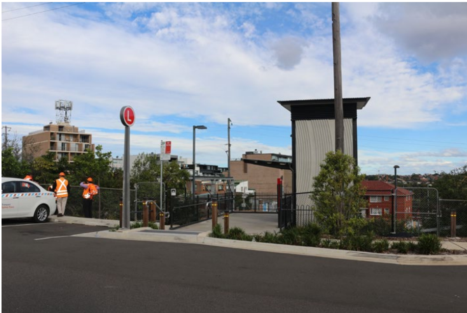
3 VIEW SOUTH FROM BEDFORD CRESCENT TO DULWICH HILL LIGHT RAIL STATION ENTRANCE
