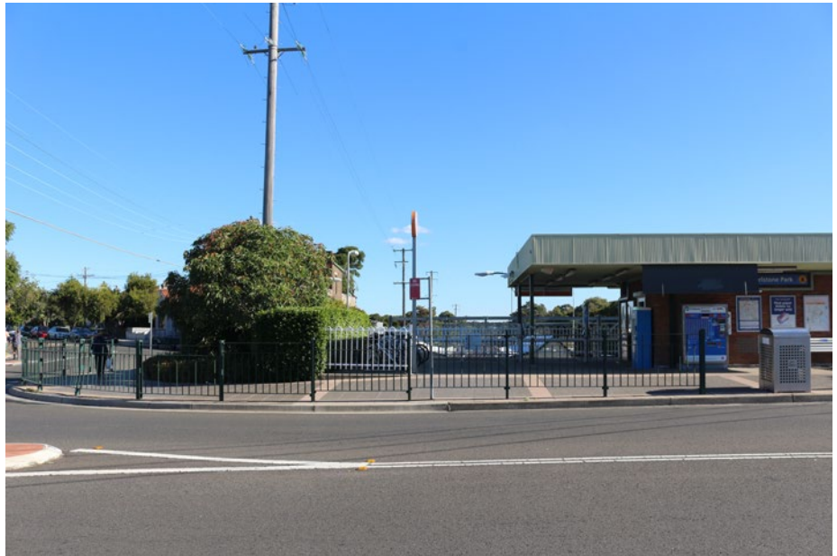
3 VIEW SOUTHWEST FROM THE FLOSS STREET RAIL BRIDGE SOUTH
