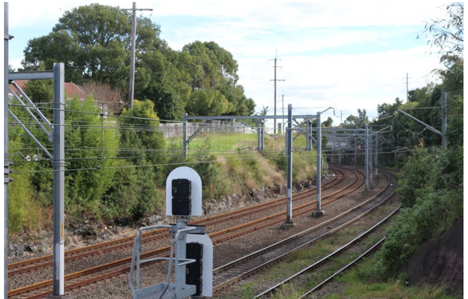
2 VIEW WEST FROM THE LIVINGSTONE ROAD RAIL BRIDGE
