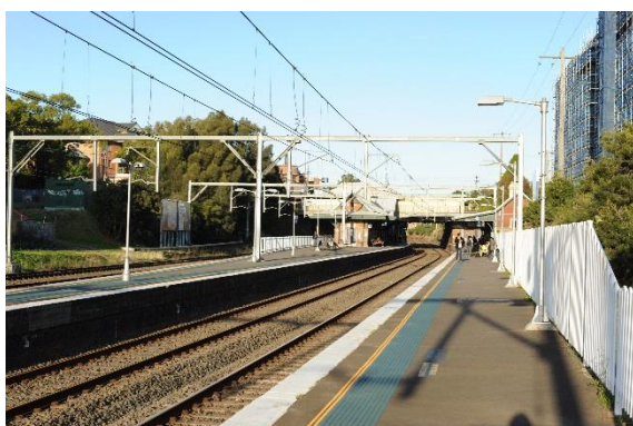
Plate 8: Canterbury Station, view east from western edge of platform three
