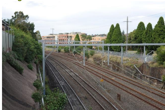
Plate 25: View east from Canterbury Road Bridge
