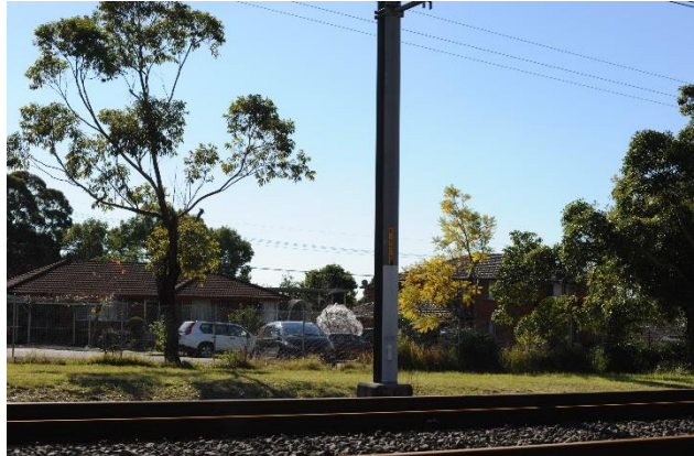
Plate 17: View north from western end of proposed construction compound. Rail at street level
