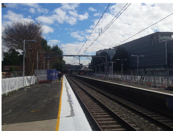
Plate 2: Marrickville Station survey unit view east
