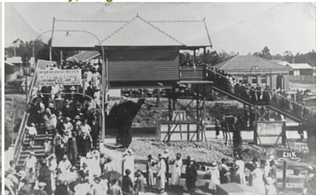
Figure 69: Opening of the overhead bridge. City of Canterbury Library Collection via Pictorial Canterbury, Image No. 30416.
