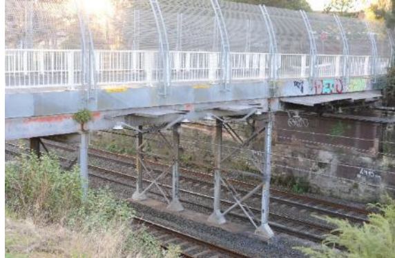
Figure 168: View of conservation area near Albermarle Street bridge, north-west aspect
