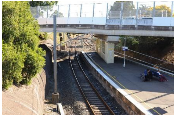
Figure 268: View of platform and overbridge, west aspect
