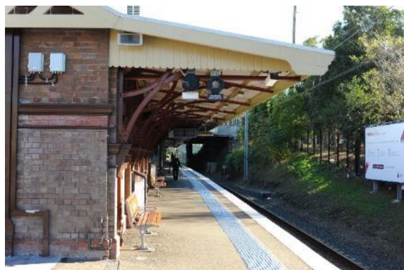
Figure 283: View of Platform 1, west aspect
