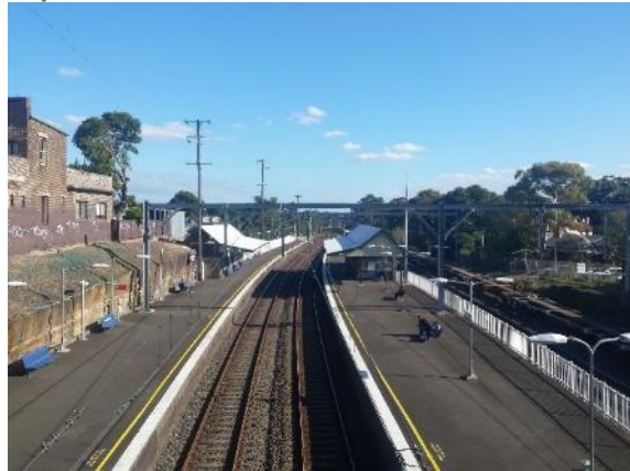
Figure 171: View of Platforms, south-west aspect
