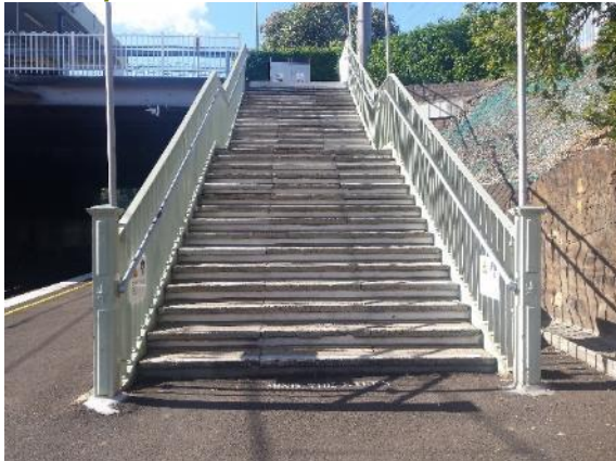
Figure 172: View of Platform 2 stairs, north-east aspect
