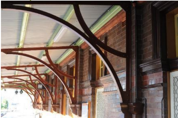
Figure 286: View of platform building detail, east aspect
