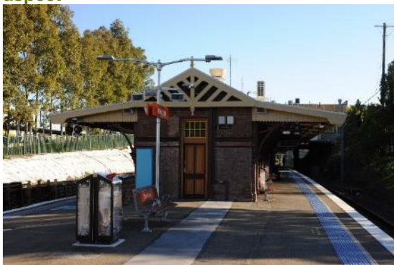
Figure 282: View of platform building, west aspect
