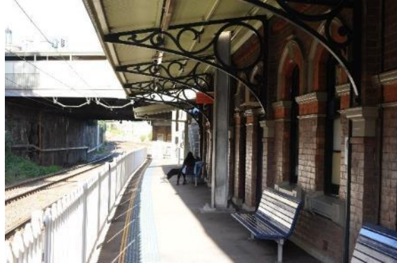
Figure 194: View of Platform 1 building detail, south-east aspect
