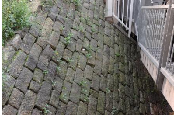
Figure 215: View of stone retaining wall, south-east aspect
