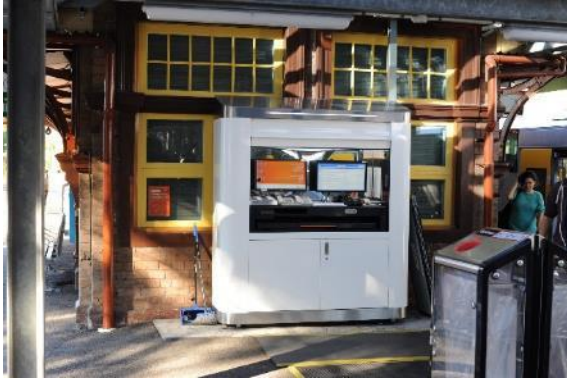
Figure 284: View of platform building, east aspect
