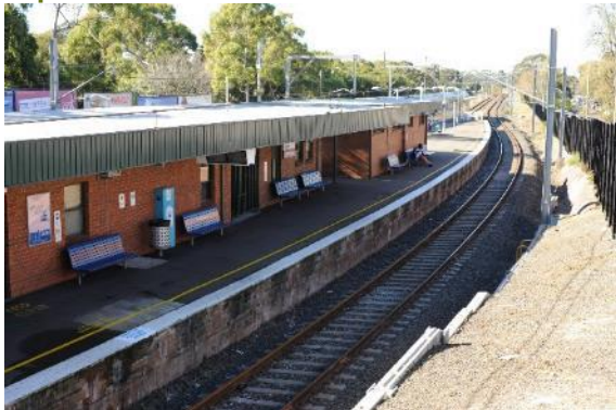
Figure 267: View of platform building, east aspect
