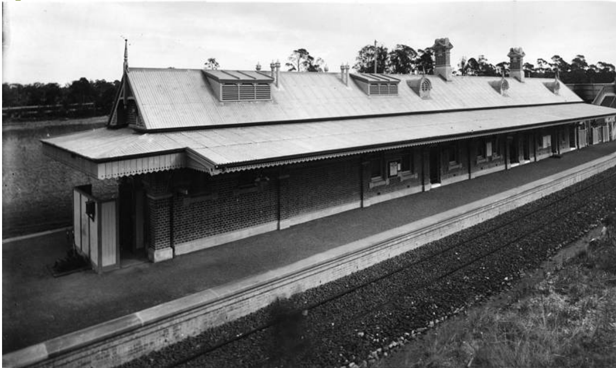
Figure 5: Belmore Station as constructed in 1890s. OEH SHI
