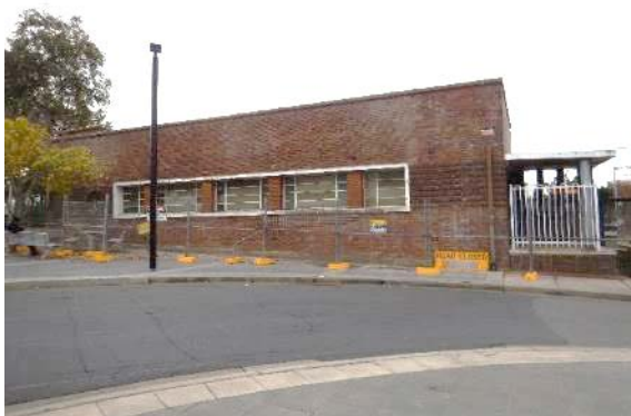
Figure 290: View of parcels office, north aspect
