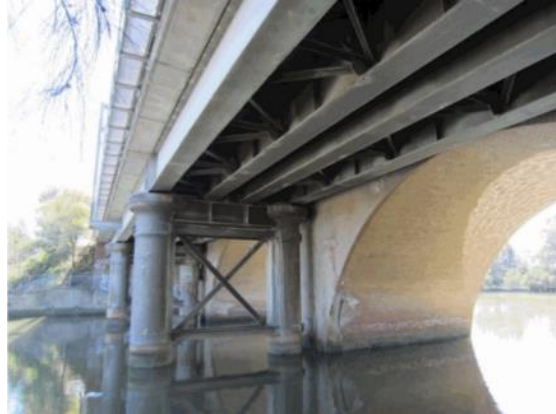
Figure 204: Close up view of underbridge structure, north-west aspect (Sydney trains)
