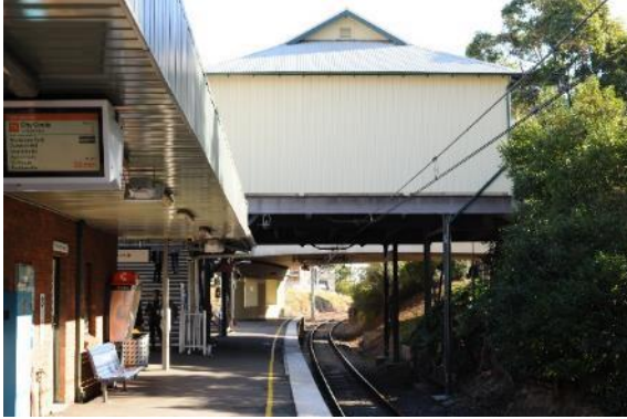
Figure 277: View of overhead booking office and Platform 1, west aspect
