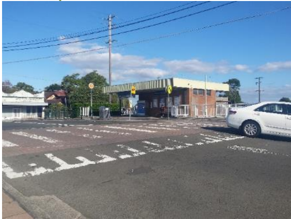
Figure 170: View of overhead booking office, south aspect
