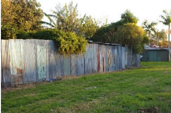
Figure 165: View of conservation area near railway corridor, south-west aspect
