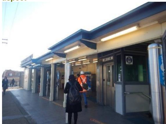
Figure 218: View of station entrance, north aspect
