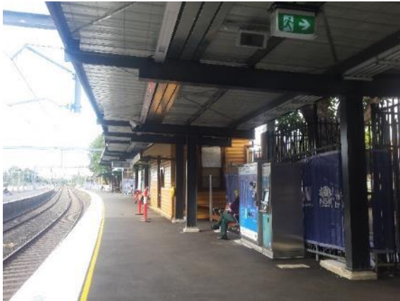
Figure 125: View of Platform 1 and 2, west aspect
