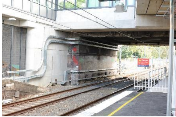
Figure 130: View of overbridge, west aspect
