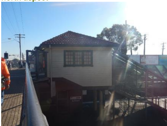
Figure 217: View of overhead booking office, north aspect
