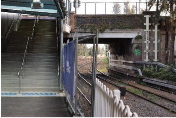
Figure 129: View of stairs and overbridge, west aspect
