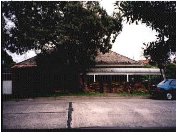
Figure 143: View of Stone house, north-east aspect (Source: OEH SHI)
