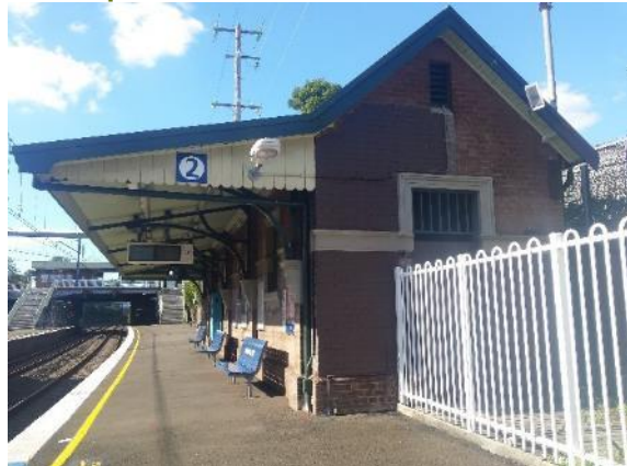
Figure 173: View of Platform 2 building, north-east aspect
