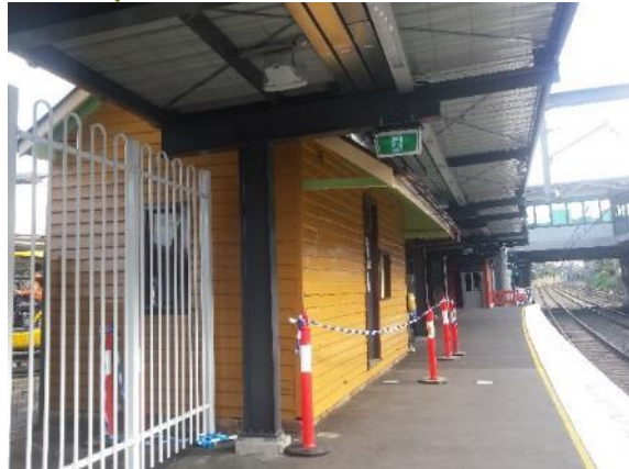
Figure 126: View of Platform 1 building, west aspect
