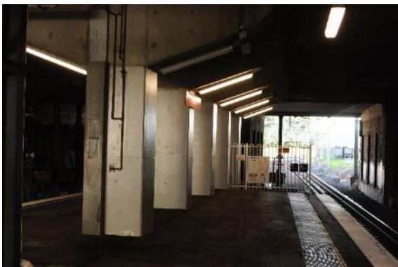
Figure 288: View of overbridge, west aspect
