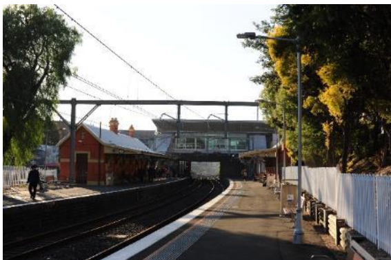
Figure 206: View of platforms, east aspect
