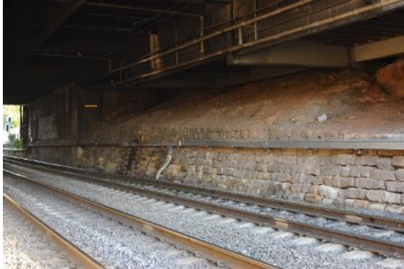
Figure 214: View of overbridge and stone retaining wall, west aspect
