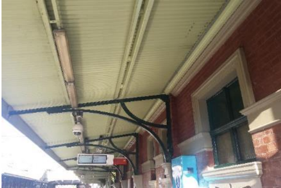
Figure 193: View of Platform 1 building, east aspect
