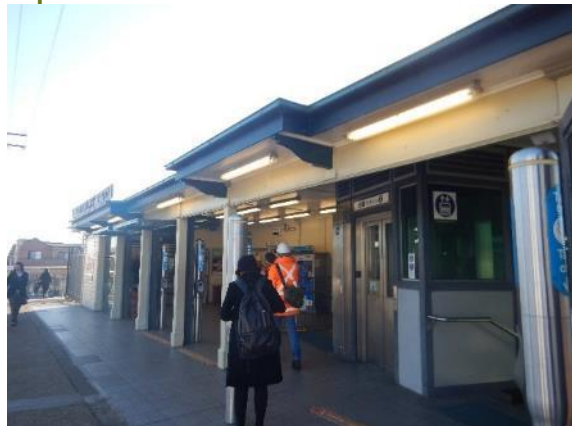
Figure 218: View of station entrance, north aspect
