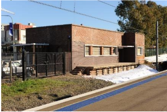
Figure 292: View of parcels office, south-west aspect
