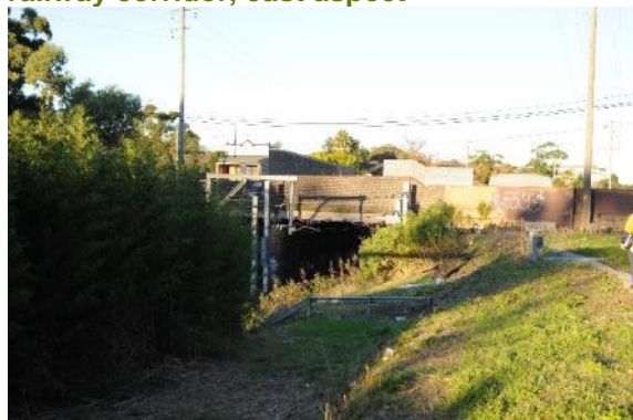
Figure 160: View of conservation area near railway corridor, east aspect
