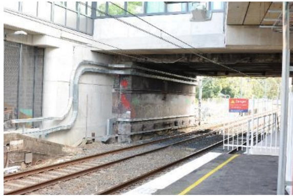
Figure 130: View of overbridge, west aspect
