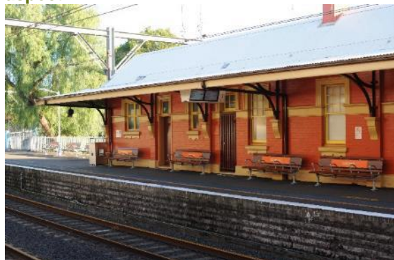
Figure 207: View of Platform 1 building, west aspect
