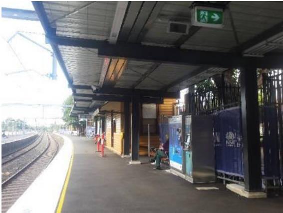
Figure 125: View of Platform 1 and 2, west aspect
