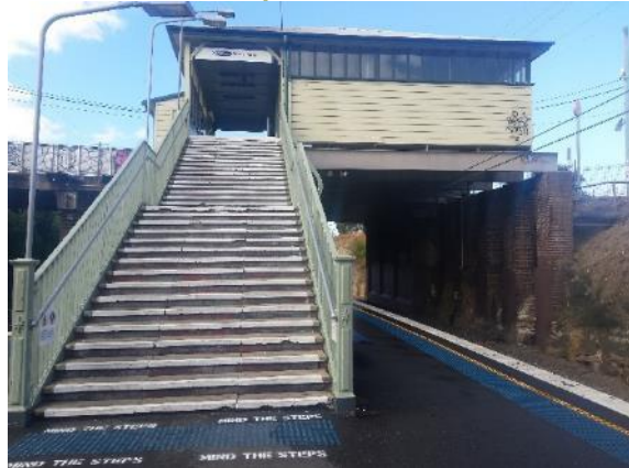
Figure 154: View of overhead booking office and stairs, east aspect
