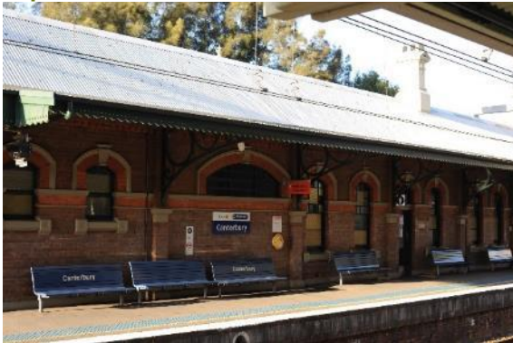
Figure 195: View of footbridge, south-east aspect
