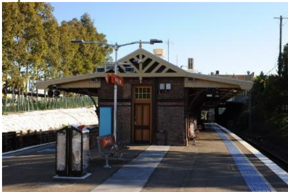
Figure 282: View of platform building, west aspect
