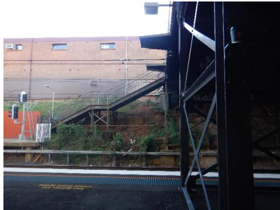
Plate 11: Campsie Station is located within a cut below street level
