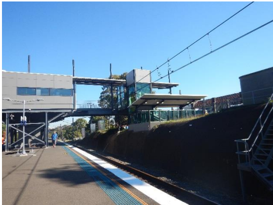
Plate 14: Lakemba Station view west along Platform 1. This image shows the shallow cut in which the station and rail is located
