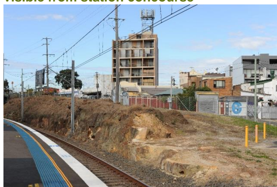
Plate 5: Underlying Hawkesbury sandstone is visible from station concourse
