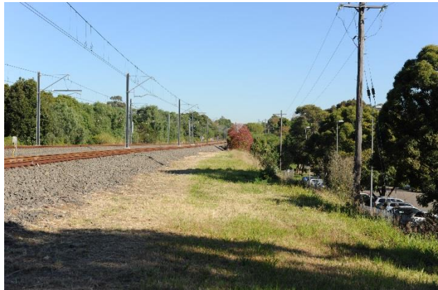
Plate 15: View west across proposed construction compound adjacent to Lakemba Station. The rail is located on an artificial embankment above street level at this location
