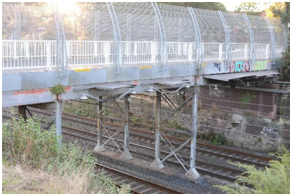
Plate 24: Albermarle Road Bridge located between Marrickville and Dulwich Hill
