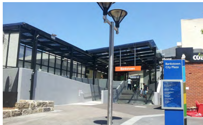
Figure 13-3: Approach to Bankstown Station
