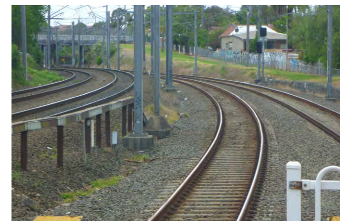
Figure 5-5: Freight and passenger rail corridors from station platform
