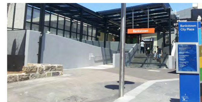
Figure 13-28: Bankstown Station Sydney Trains northern entry
