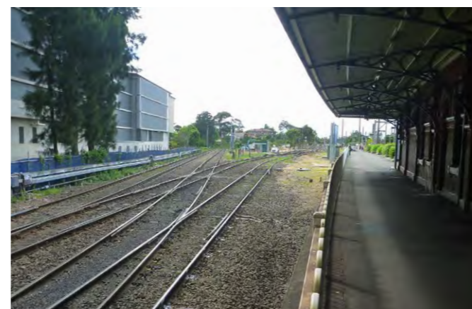
Figure 4-4: View of rail corridor
