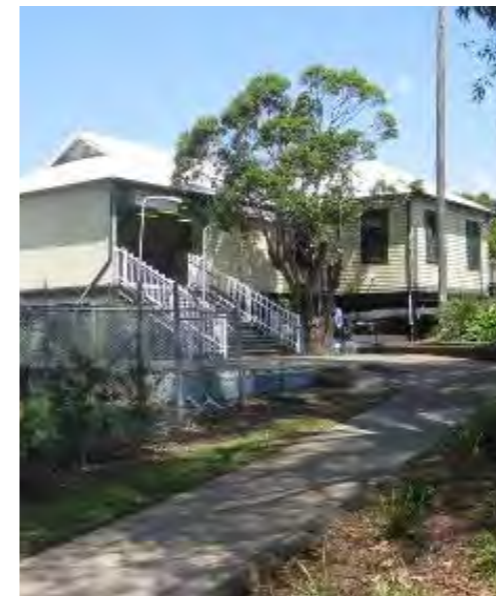
Figure 12-10: Punchbowl Station Booking Office Source: OCP Architects
