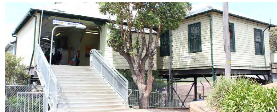
Figure 12-13: Punchbowl Station northern entry
