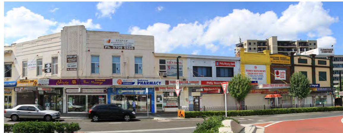
Figure 13-12: Bankstown Town Centre Source: Adam J.W.C
