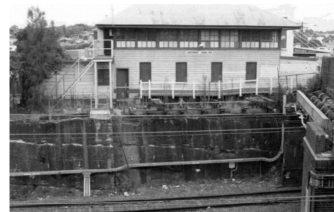
Figure 7-9: Canterbury Station Signal Box Source: NSW Government
