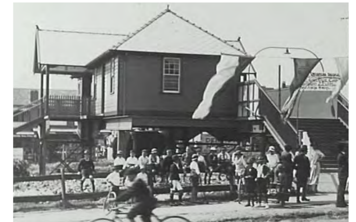
Figure 10-8: Lakemba Railway Station 1926 Source: City of Canterbury
