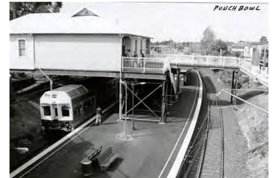
Figure 12-11: Survey of Railway Footbridges Source: State Rail Authority
