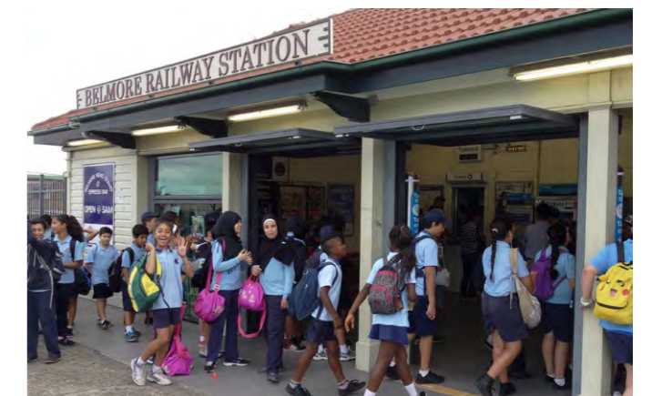
Figure 9-31: Existing station entry
