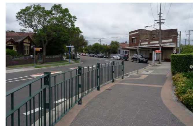
Figure 6-27: Duntroon Street - southern side of station
