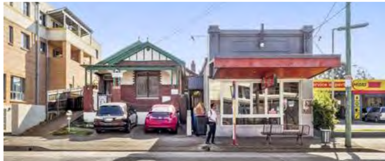
Figure 8-13: Beamish Street, Campsie Source: Commerical Real Estate
