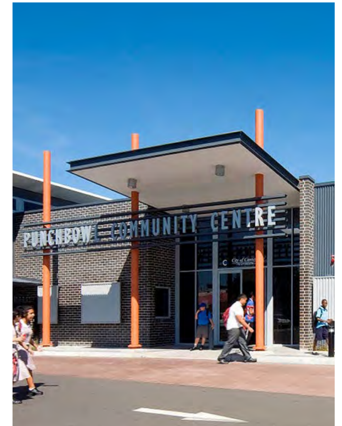
Figure 12-19: Punchbowl Community Centre Source: GroupN
