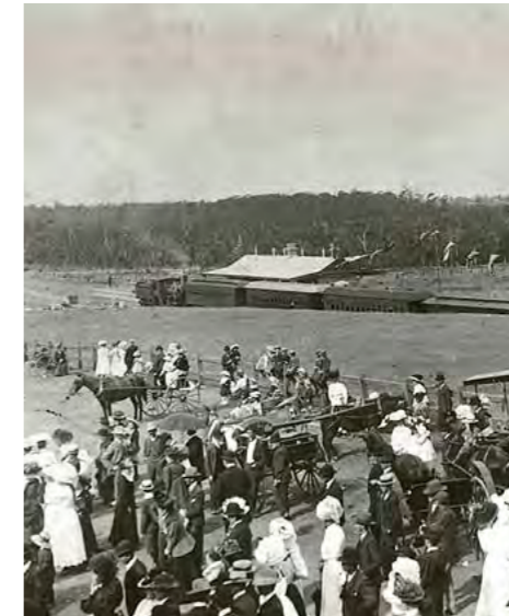
Figure 13-7: Bankstown Station Opening 1909 Source: NSW State Government
