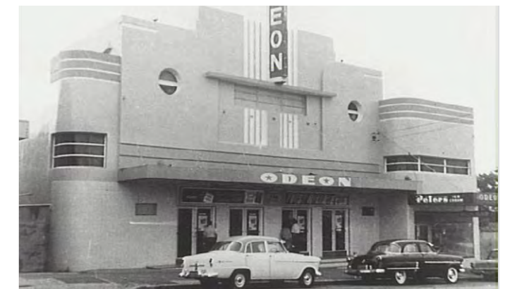
Figure 10-9: Odeon Theatre 1960s Source: City of Canterbury
