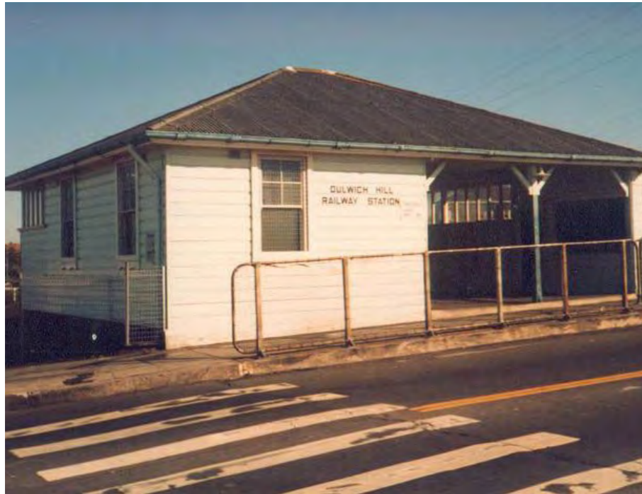
Figure 5-9: Overhead Booking Office, 1985 Source: NSW Government
