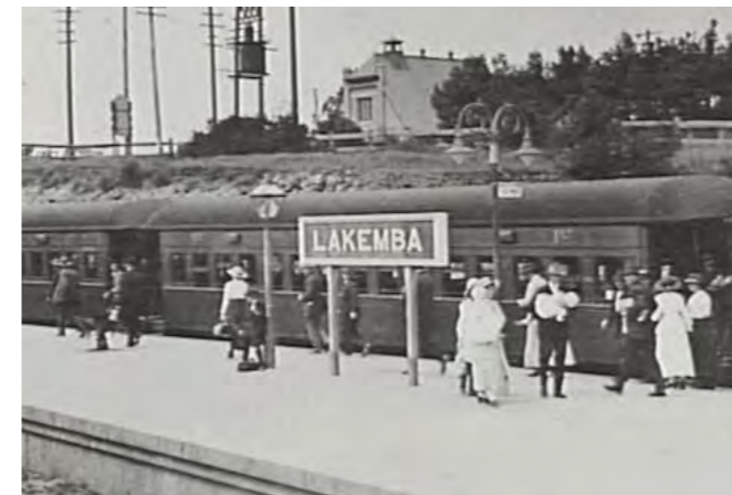
Figure 10-7: Lakemba Railway Station 1910 Source: City of Canterbury
