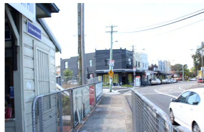
Figure 5-4: Wardell Road bridge footpath
