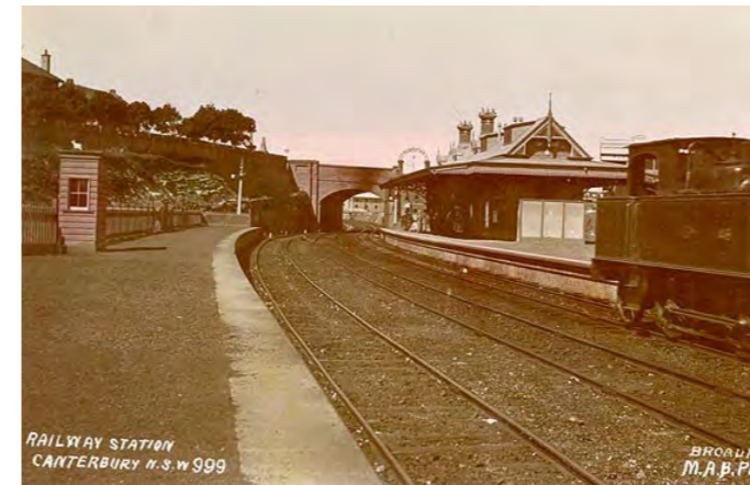
Figure 7-7: Canterbury Station 1916-1926 Source: NSW Government
