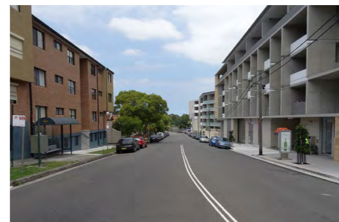
Figure 4-28: Contemporary development adjacent to Marrickville station
