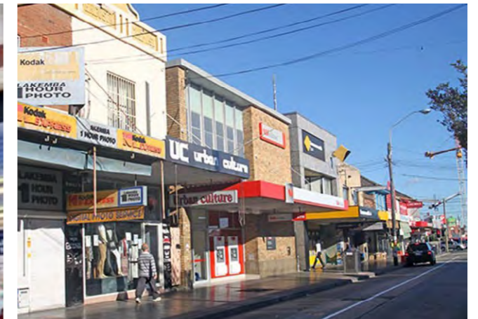
Figure 10-13: Haldon Street retail/commercial strip
