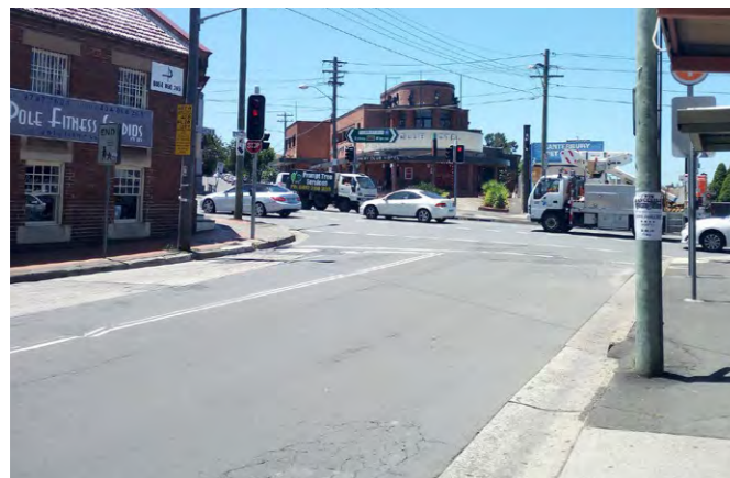
Figure 7-28: View from Broughton Street to Canterbury Road
