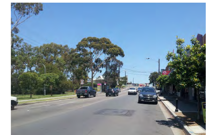
Figure 12-30: Site of proposed crossing on Punchbowl Road
