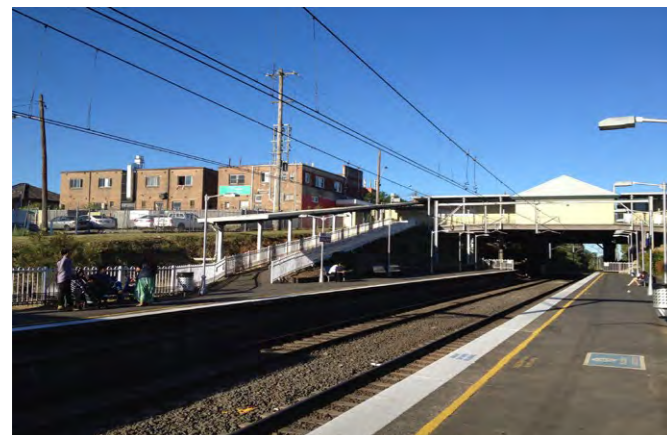
Figure 11-24: Wiley Park Station concourse from platform
