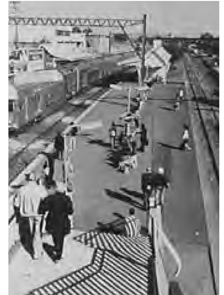
Figure 8-9: Campsie Railway Station Source: Canterbury City Council
