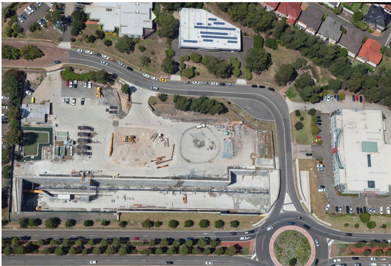
Figure 3 - Aerial View of the Sydney Metro Norwest Station Site
