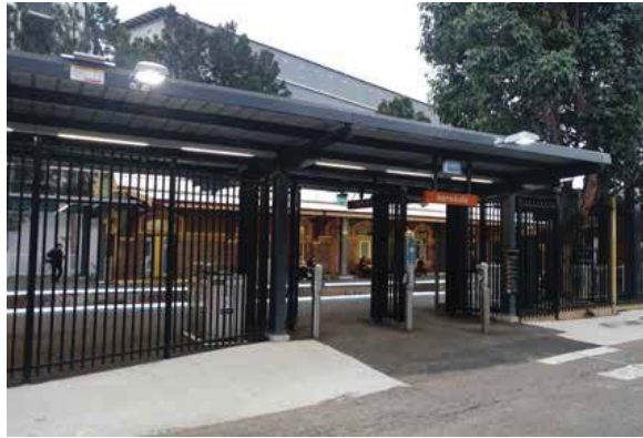
Existing Station Street entry Source: COX/HASSELL
