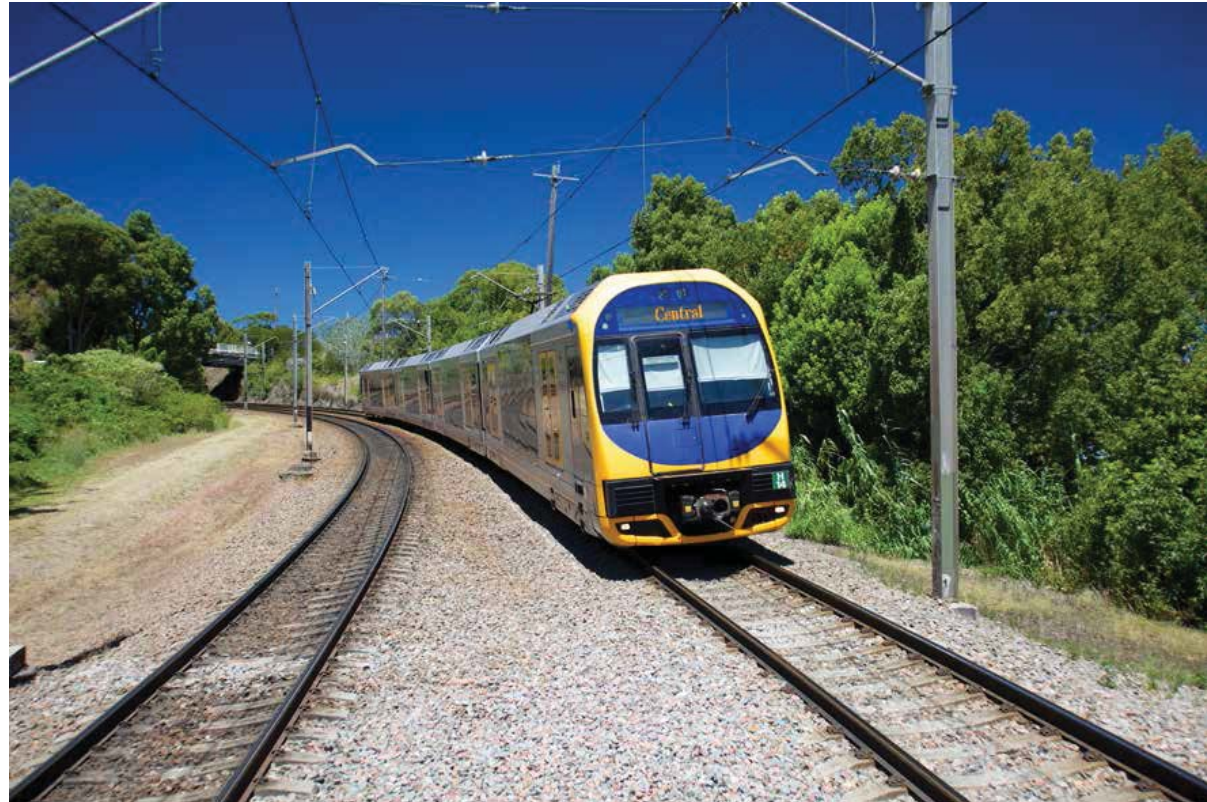
Rail Corridor with Sydney Trains service Source: TfNSW, Photographer: Simon Freeman 2013
