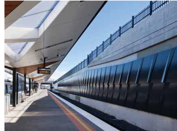
South Morang Station, Vic. Services are rationalised, integrated into retaining wall design.
