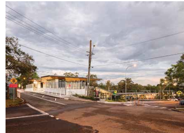
Cheltenham Station Source: COX
