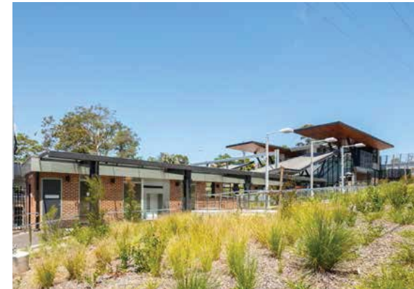
WSUD initiatives integrated at Cheltenham Station. Source: COX
