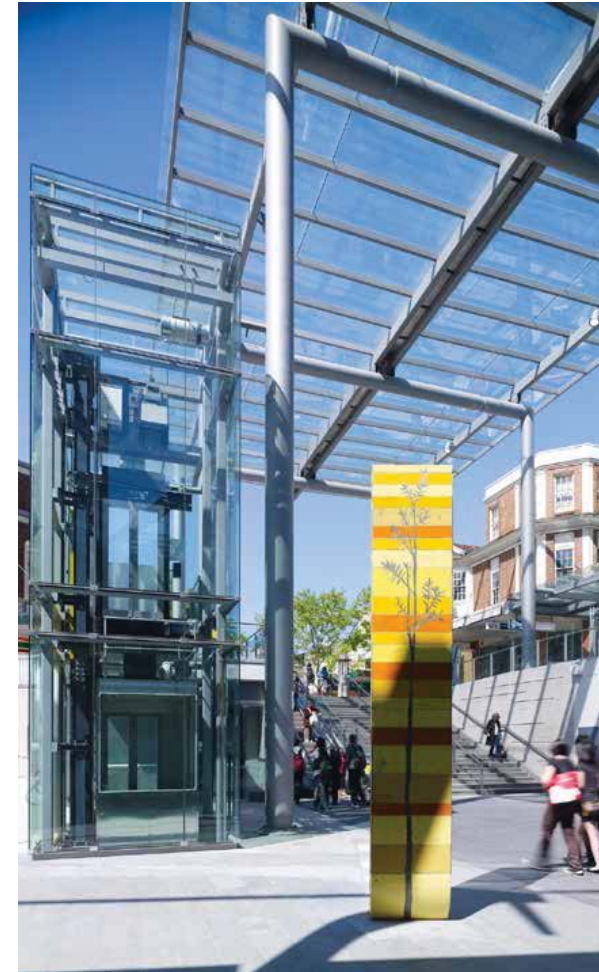
Chatswood Transport Interchange, NSW. Good example of a glazed lift and shaft Architect: CoxDesignInc. Source: COX
