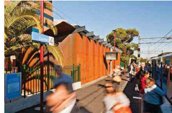
Caulfield Station, VIC. Platform service building Source: Lovell Chen
