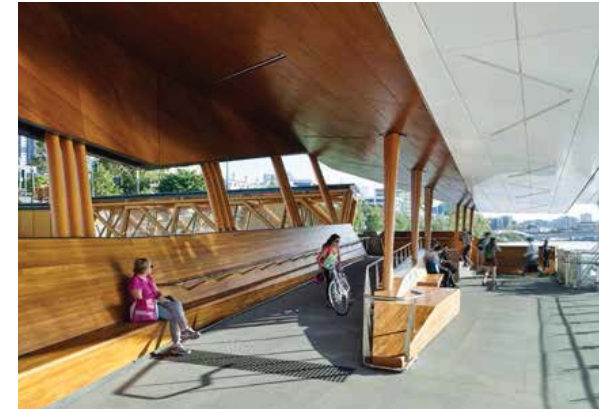
Milton Ferry Terminal, QLD. Ramps provide equal access for all customers. Integrated seating provides rest points along paths of travel. Source: COX, Copyright: Chris Frederick Jones
