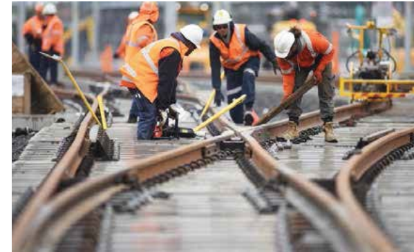
Construction of Sydney Metro Northwest. Source: TfNSW
