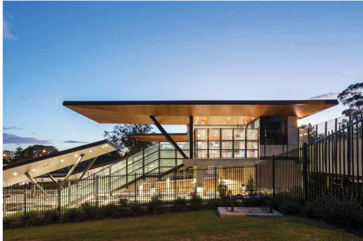
Cheltenham Station Source: COX
