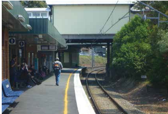
Punchbowl Station platform Source: COX/HASSELL
