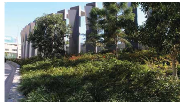
Inner Northern Busway, Brisbane. Ensure earthwork batters sit lightly in their context, exhibiting a 'natural fit' with their landscape contexts. Source: AECOM
