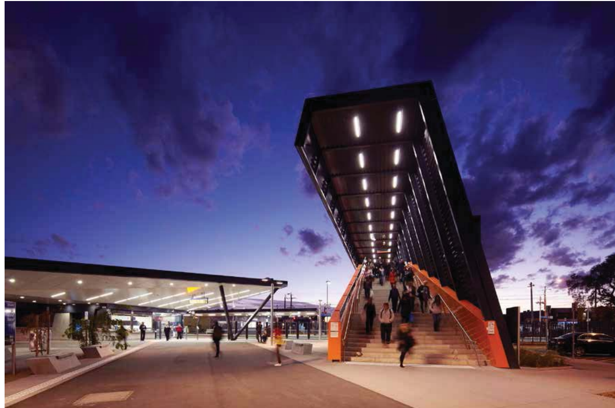
Thomastown Station, VIC. Legible station entry integrated with the public domain. Source: COX
