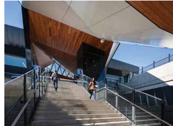
South Morang Rail Extension, VIC. Calm and neutral materials with integrated services. Source: COX
