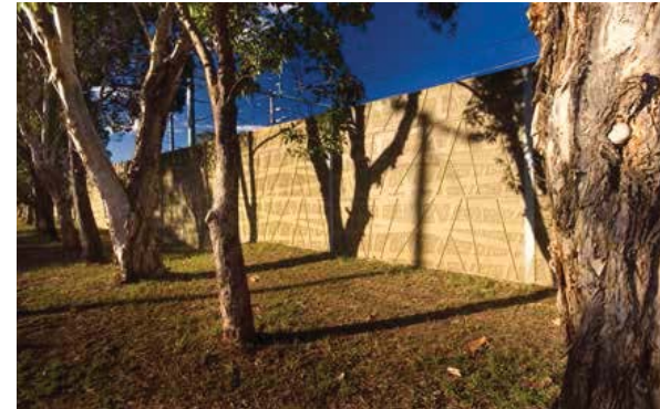
Graceville Rail Corridor, NSW. Noise Walls Source: AECOM.
