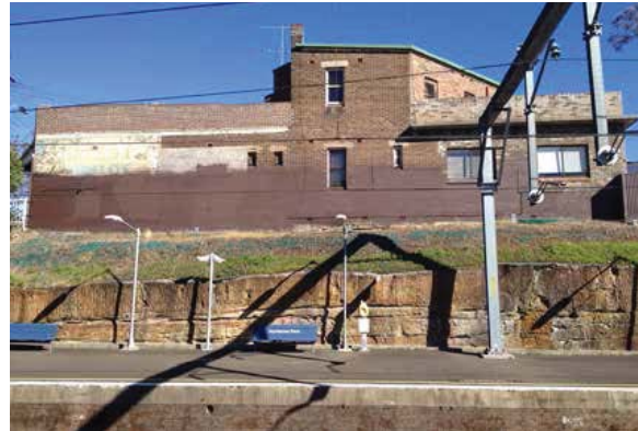
Excavated sandstone cutting on Platform 2 Source: COX/HASSELL
