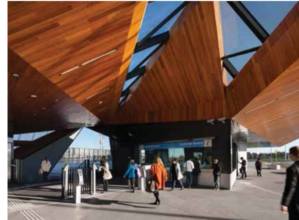
South Morang Rail Extension, Vic. Clear sight lines and circulation paths through station entry. Source: COX, Copyright: Dianna Snape
