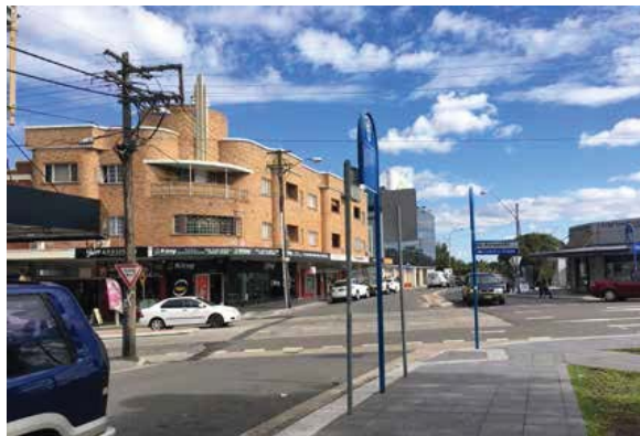
Existing buildings, Burwood Road Source: COX/HASSELL
