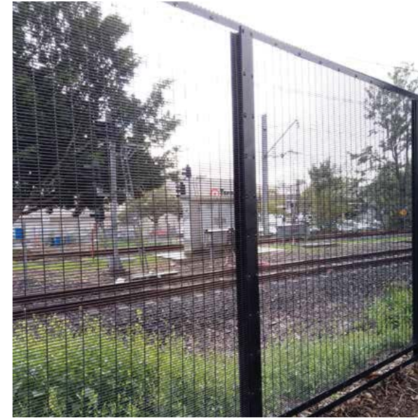
Homebush, Sydney. Rail corridor security fences should be robust, easily maintained, modular systems that are readily integrated with other urban design elements such as retaining walls. Source: COX/HASSELL
