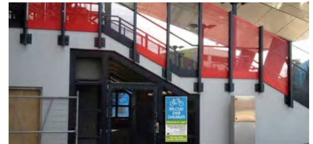
Figure 12.4 Syndal Station Melbourne (example of secure access bicycle parking facility integrated into station building under stairs)
