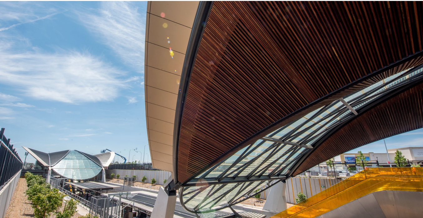
Station canopy at Bella Vista Station.
