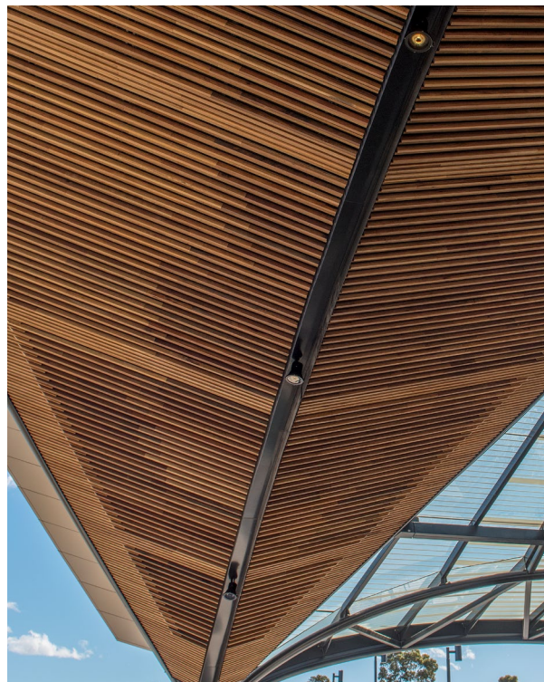
The station canopy at Norwest Station.
