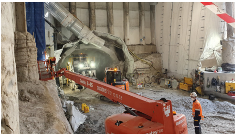
Ventilation Dust Extraction Systems placed at the face of the works.
