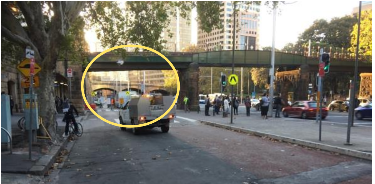
Figure 5 – Sydney Light Rail Construction Site
