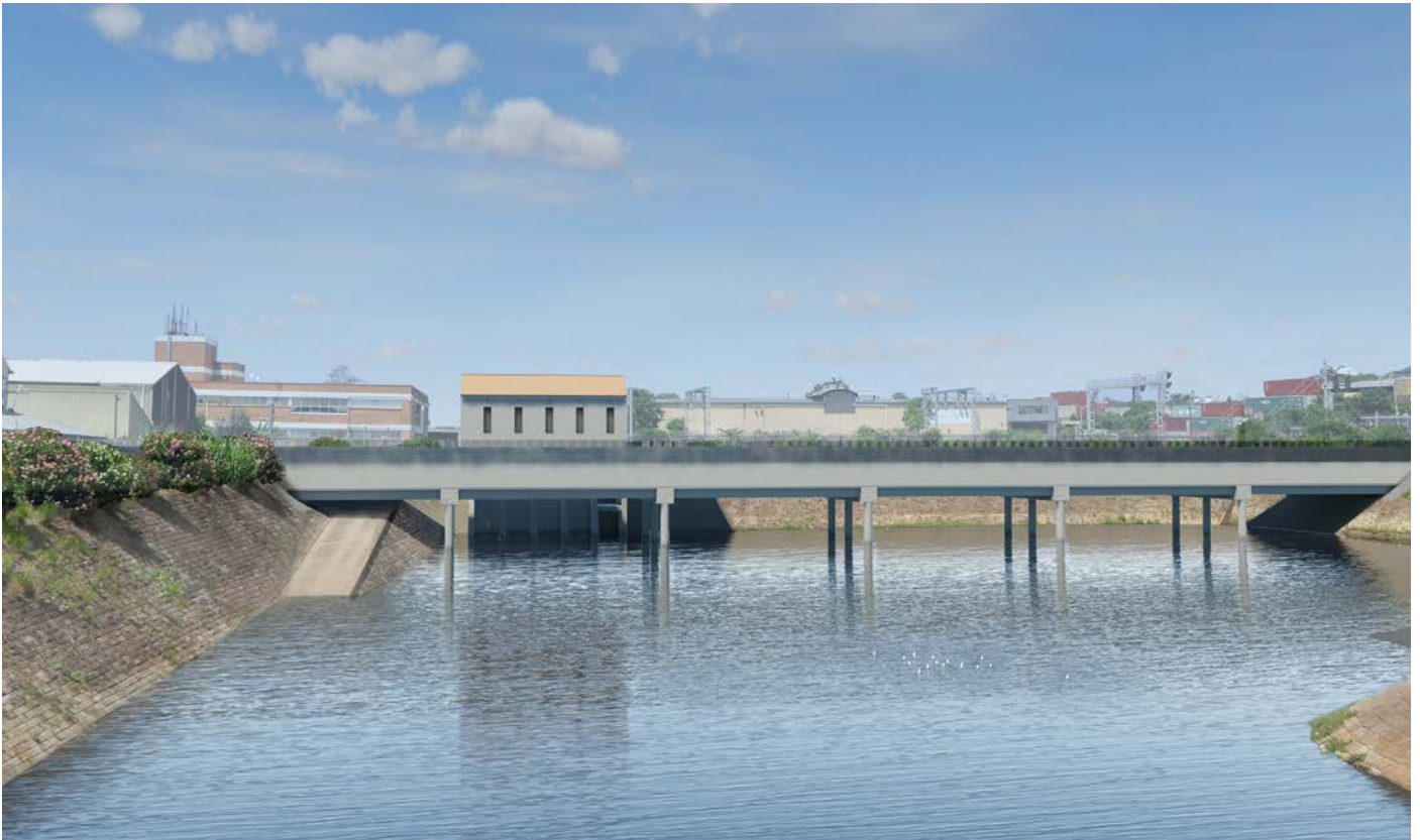
Fig 4 - Views to the Pit and Pumping Station. Source: HASSELL+WW
