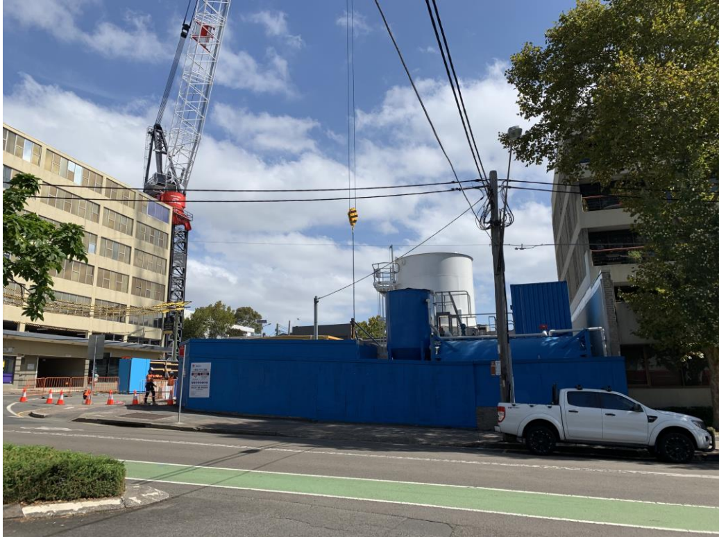
Figure 11: Current site conditions – March 2021
