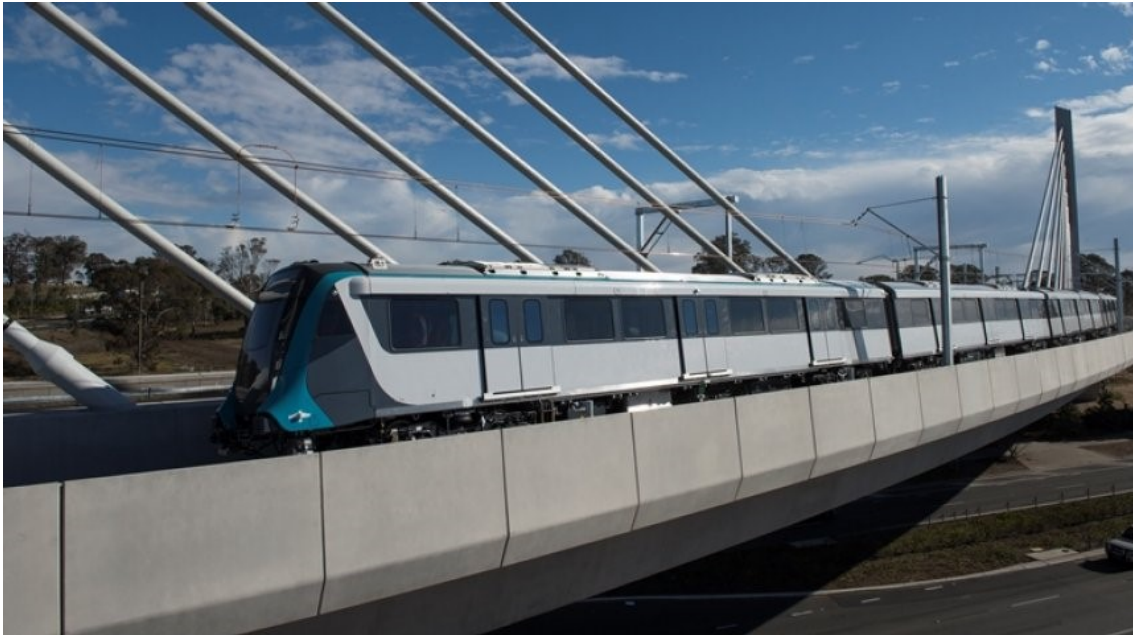
Figure 4-1 Photograph of a train operating on Sydney Metro Northwest
