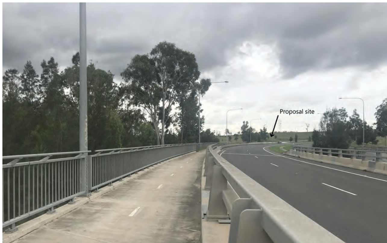
Figure 8-12: Viewpoint 4 – View north-east from Lenore Drive at the Ropes Creek crossing
