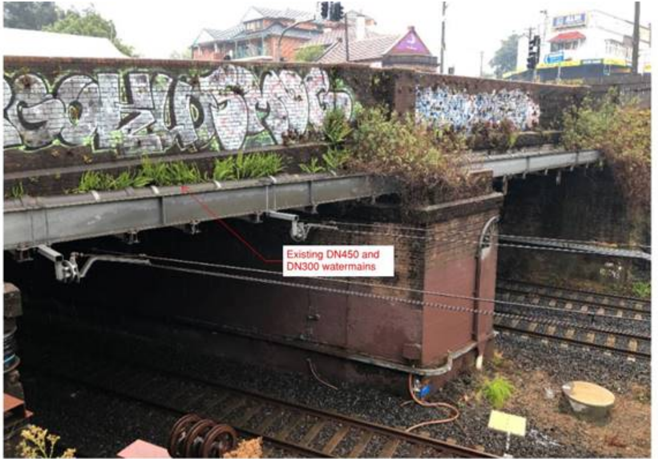
Figure 2: Canterbury Overbridge eastern side facing north at street view.
