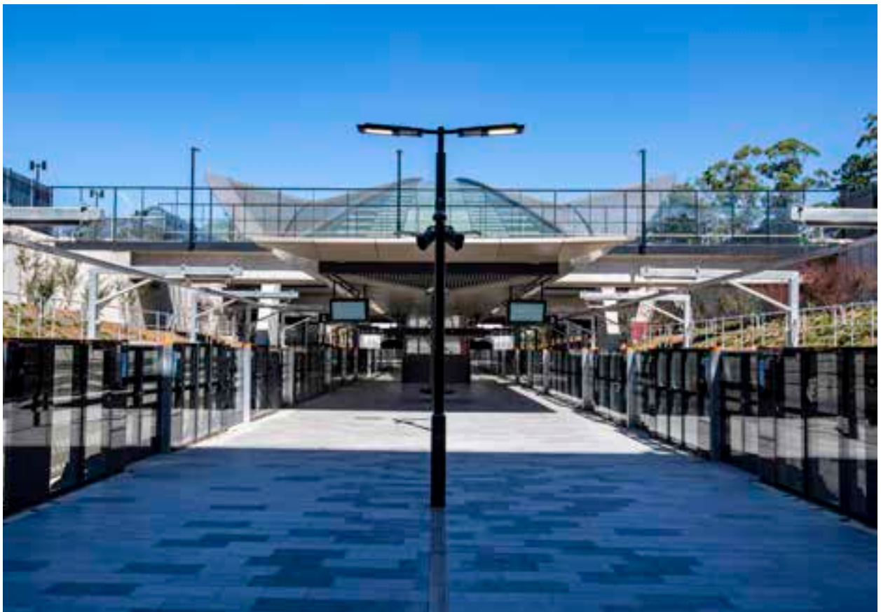
Figure 2: First look at Cherrybrook Station, February 2019.
