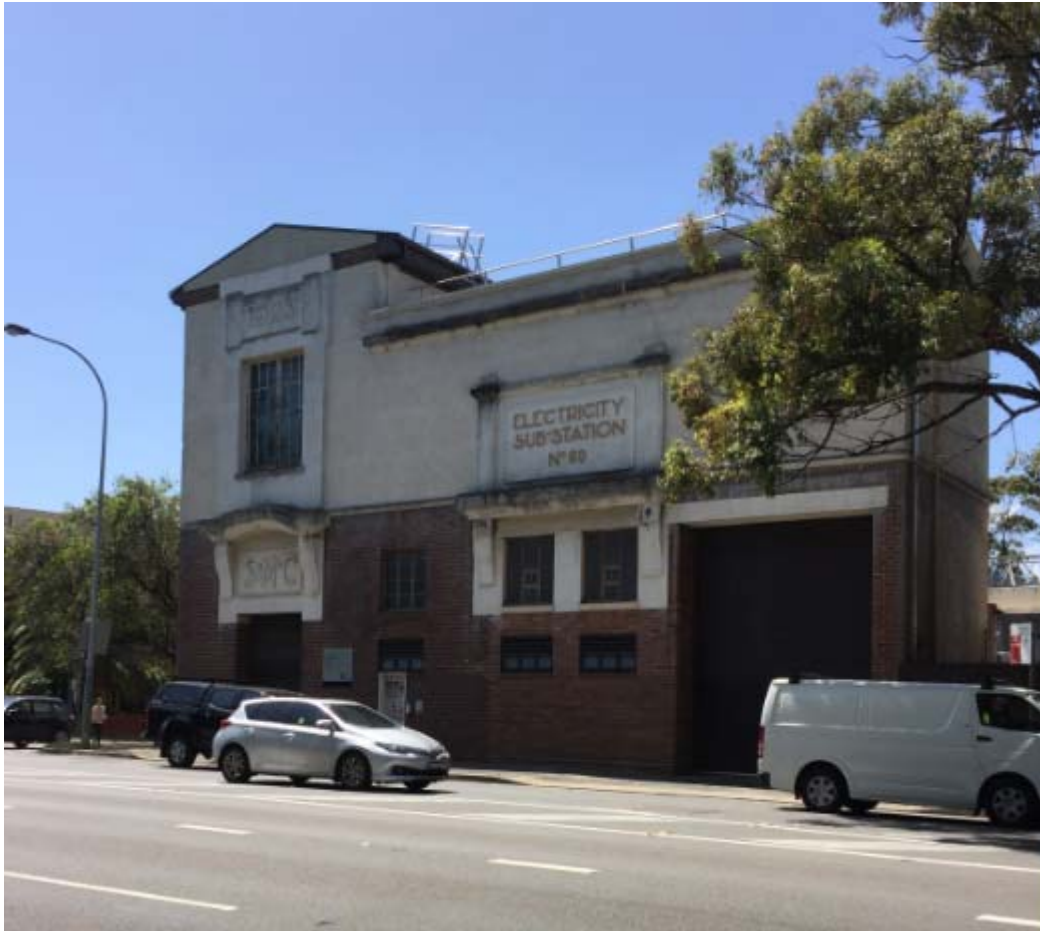
Plate 6 : Chatswood Zone Substation No. 80, looking south east (RPS, 2016).
