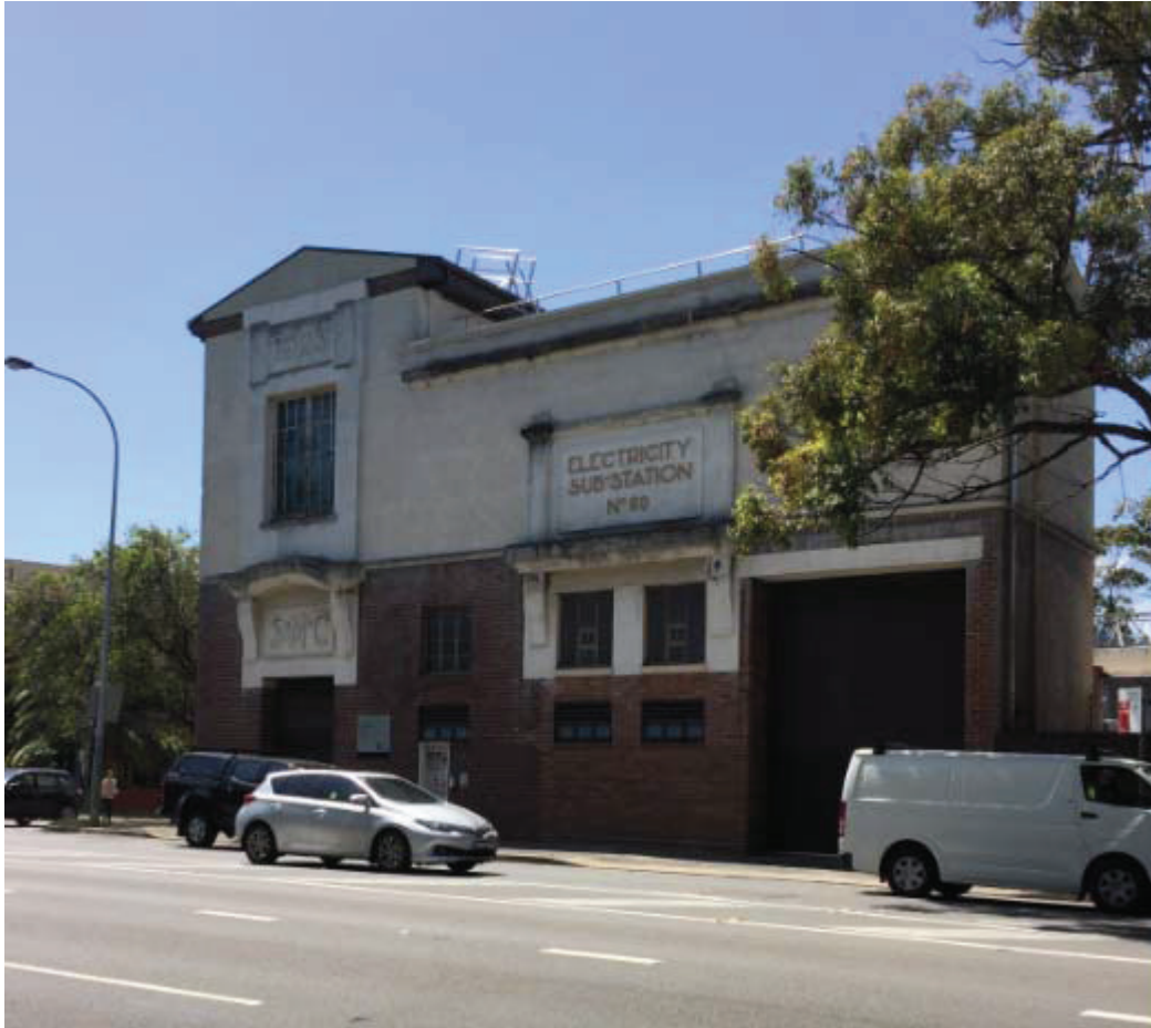
Plate 6 : Chatswood Zone Substation No. 80, looking south east (R S, 2016).
