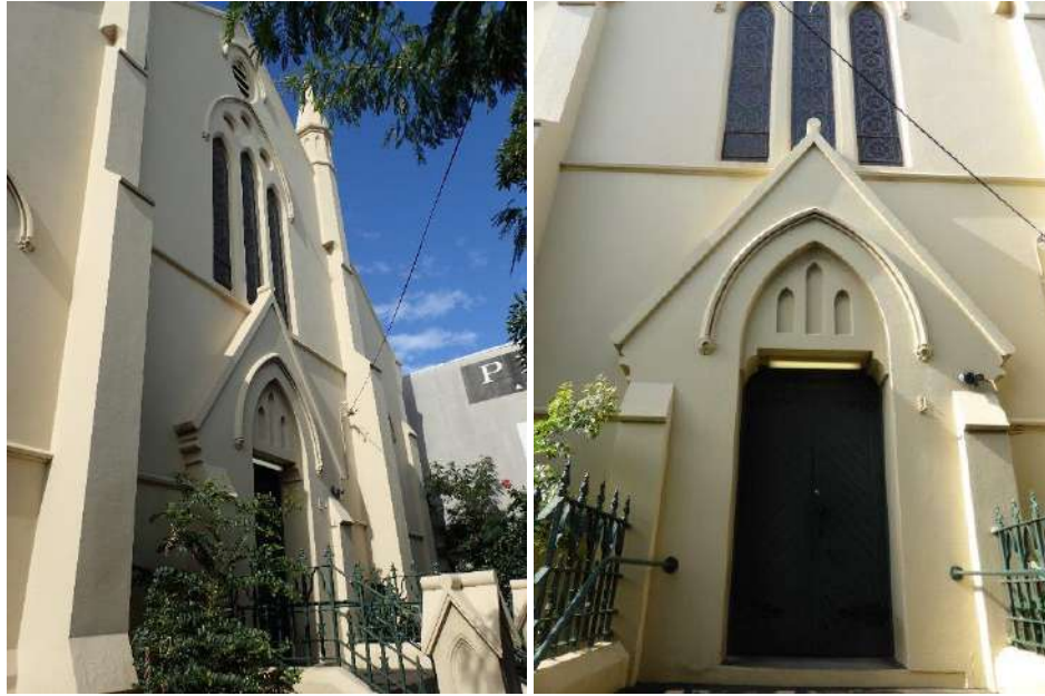
Figure 3 The entrance to the Congregational Church.
