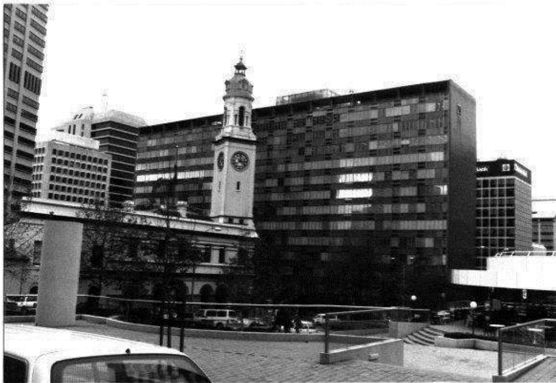
Figure 3 View of the western façade of the MLC Building (Source: North Sydney Council).
